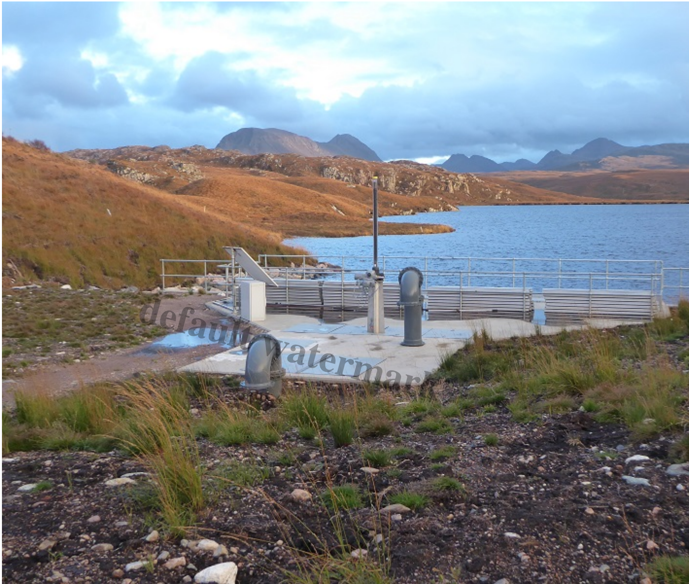
Intake to Badachro hydro scheme, with Baosbheinn and Ben Alligin behind. There is also a dam. Photo taken in Oct 2018 2 years after completion
