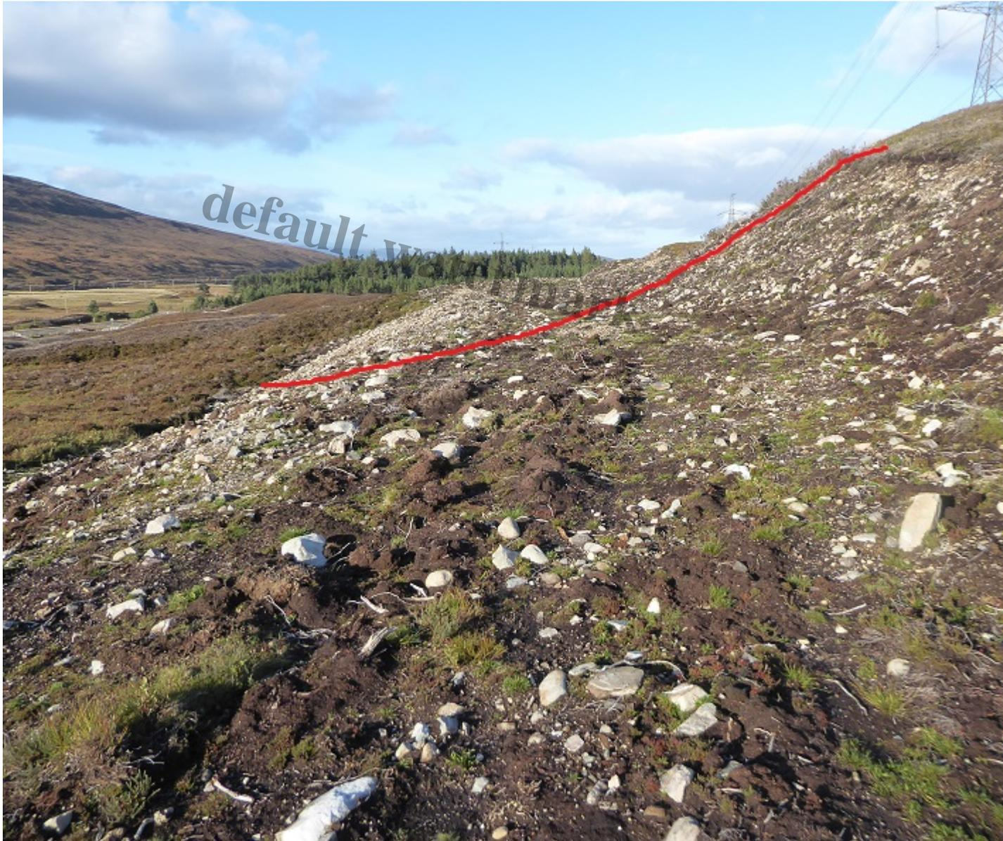
The red line is my attempt at depicting how the profile of this section of slope might have looked BEFORE the track was constructed. A great shelf has been cut across the hillside and the track constructed using the fill technique the fill being the material above the red line. Oct 2018.
