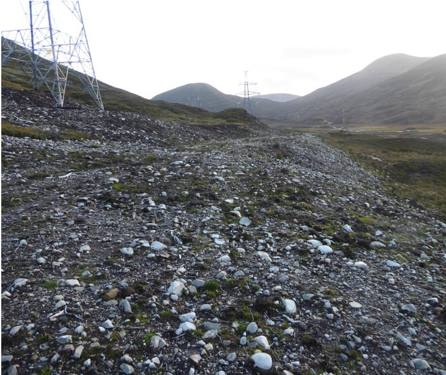
Another illustration of how spoil from the cut was moved to the moor below to create the track line. C
