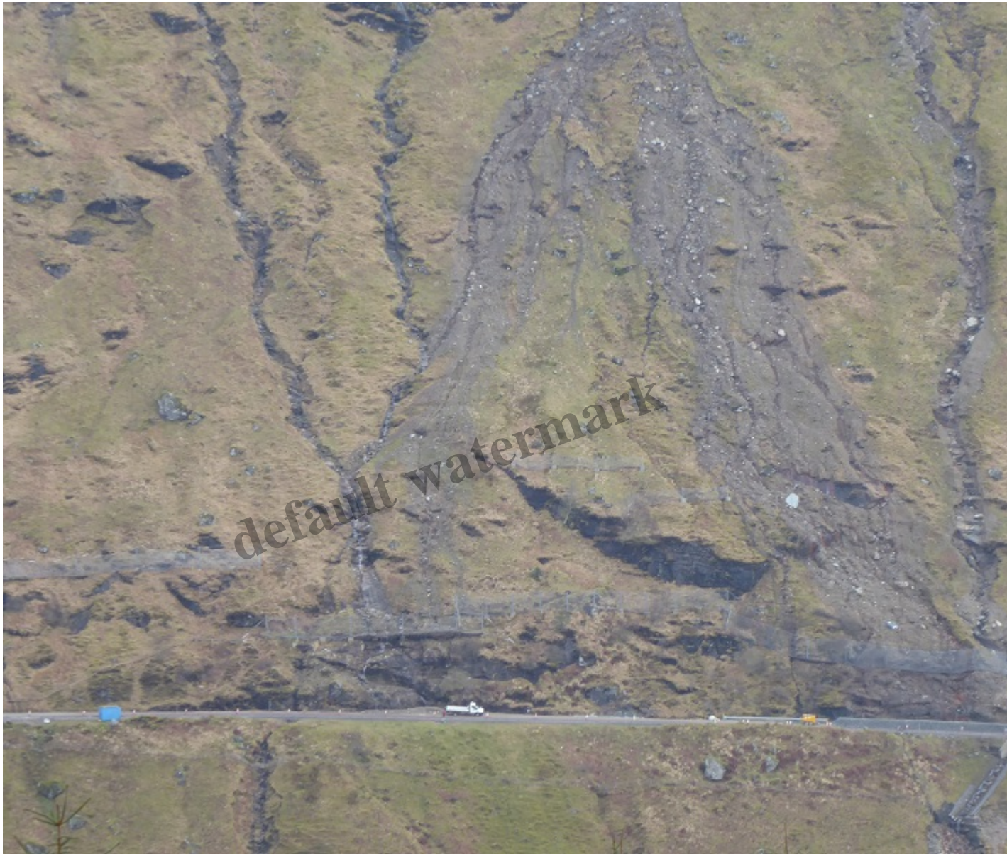
Photo illustrating volume of debris flows compared to the size of the netting
