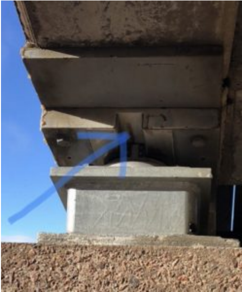
Example of bearing designed only to allow longitudinal movement – along the groove
