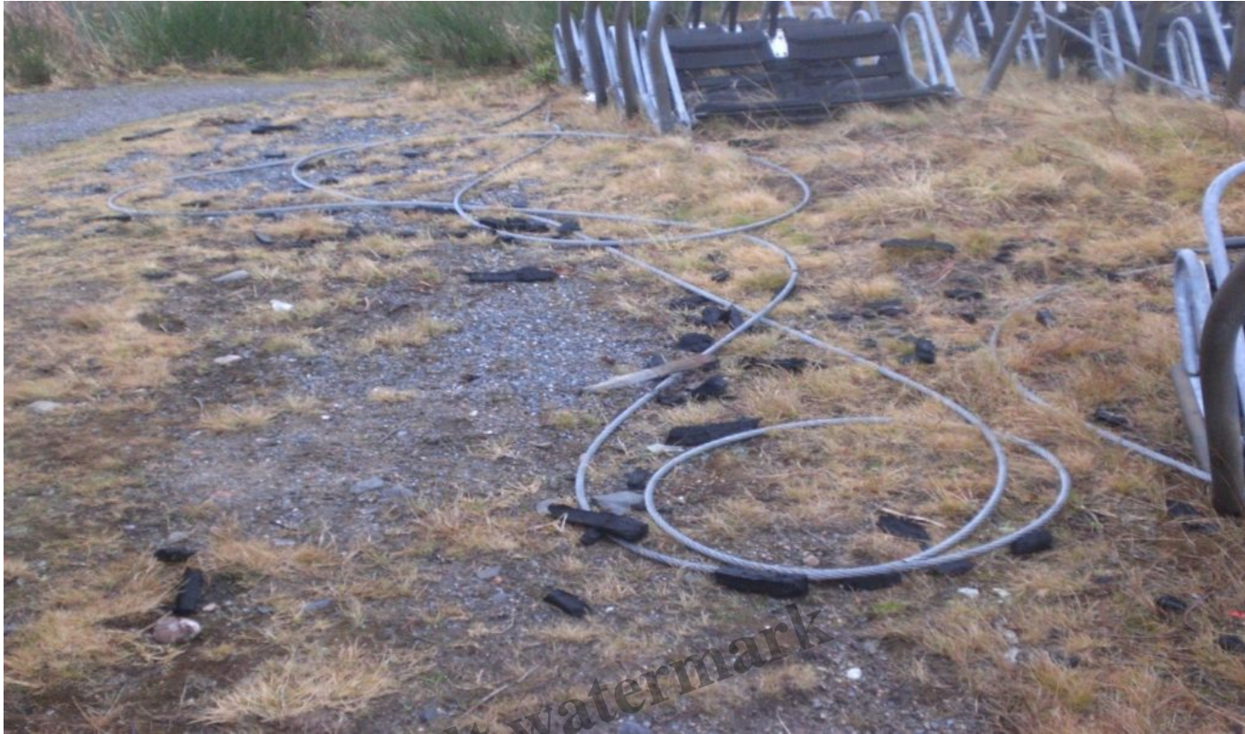
Perished rubber from the Chair seats, strewn around the area.
