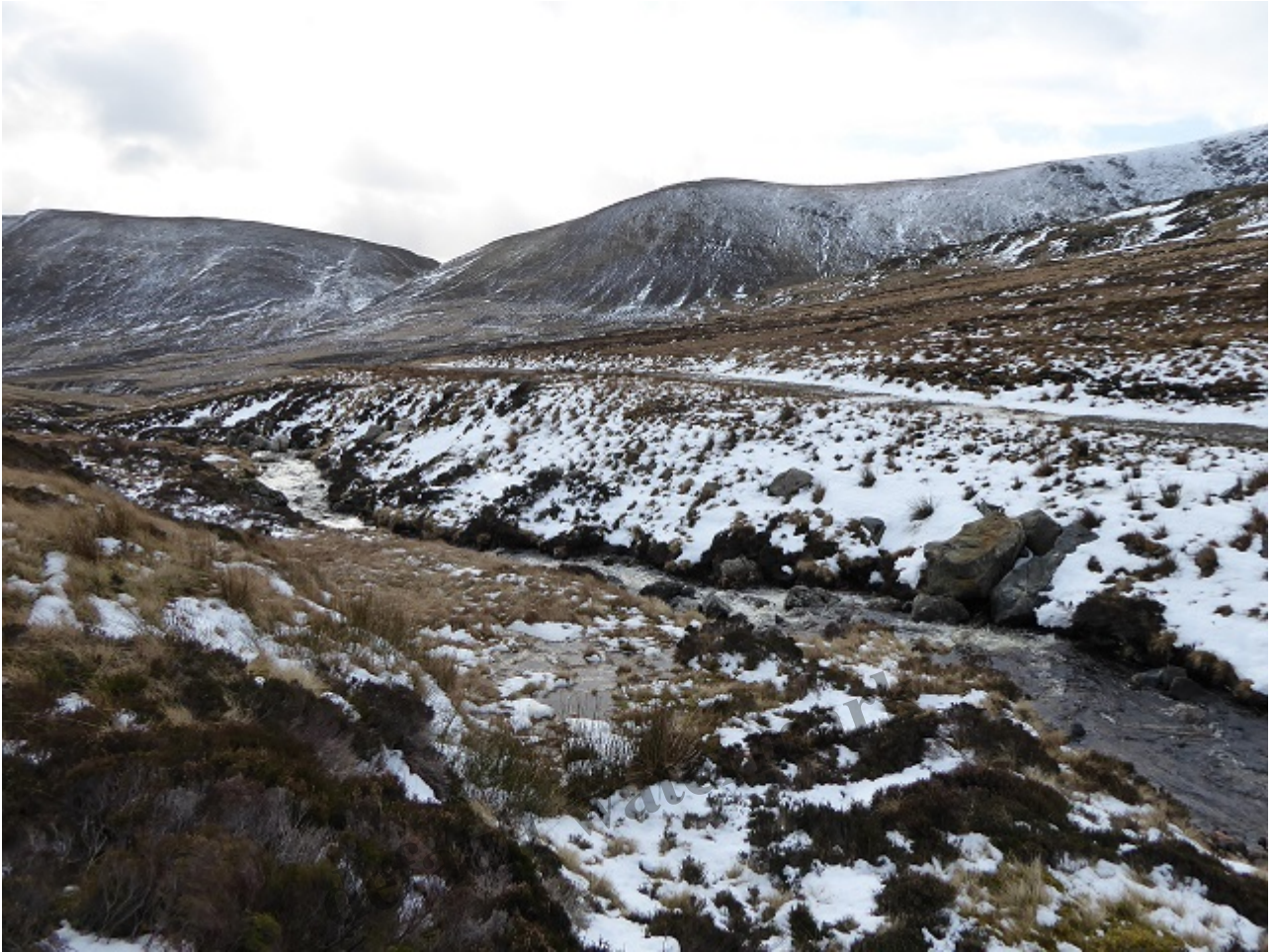
View of the road up to the Mayar intake above where it crosses the burn
