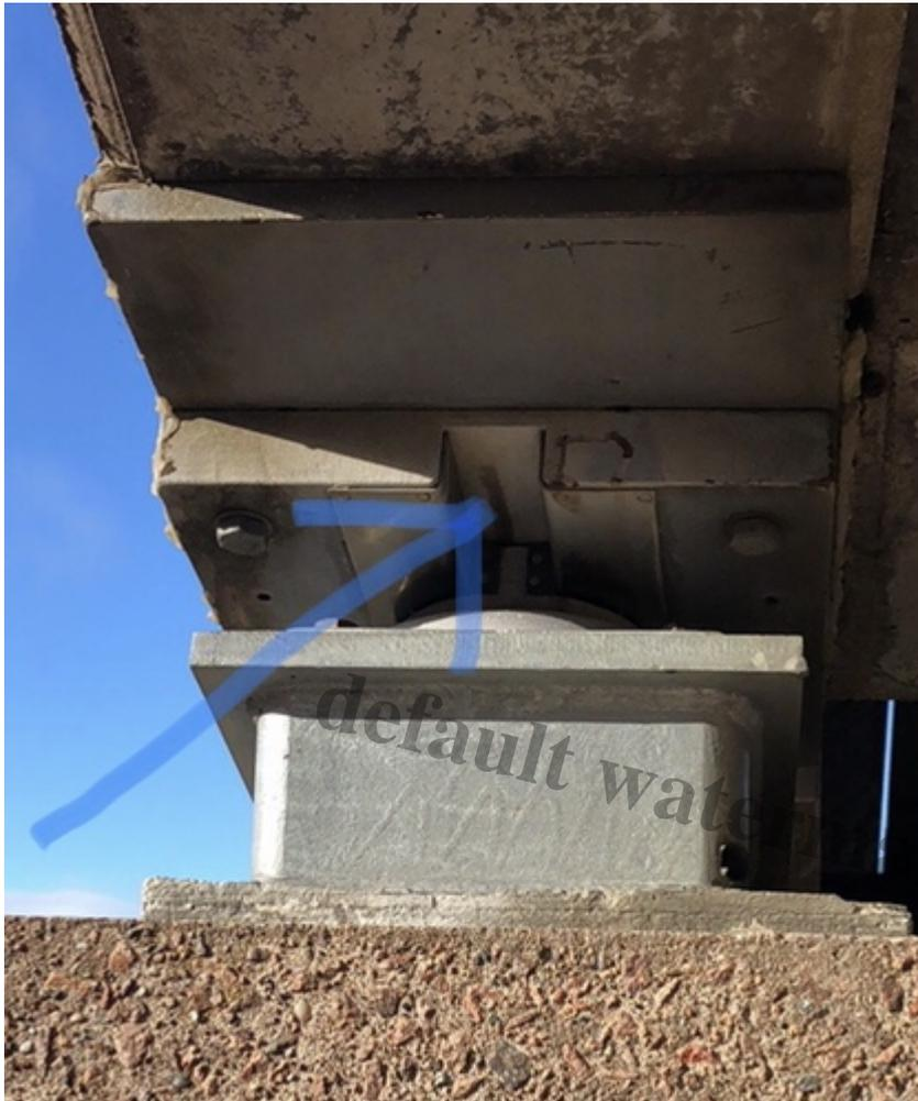
The groove with the line inside marked by the arrow showing the extent of movement along it – in this case, the movement appears to have been within normal tolerances
