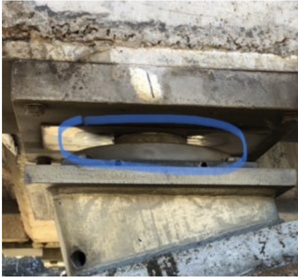
Aligned bearing
