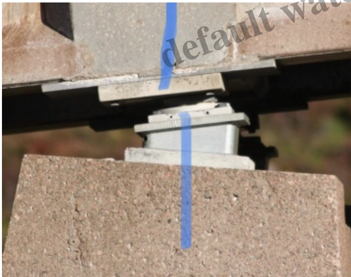
Unaligned bearing
