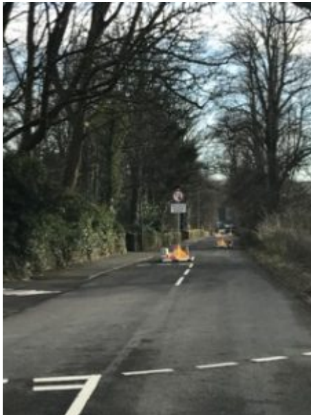
New traffic calming on the Old Luss Road
