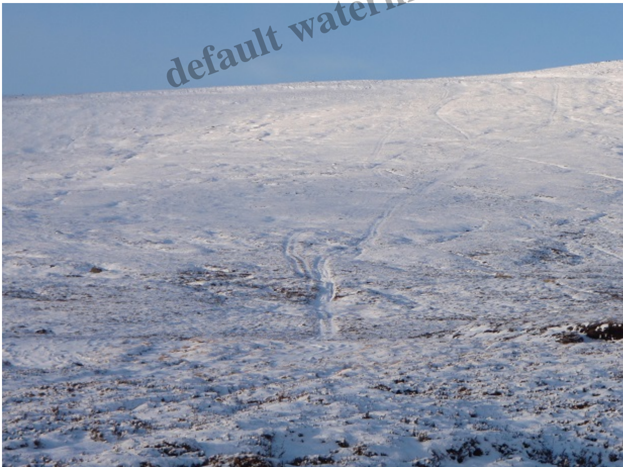
A multiple set of ATV tracks branching off the existing hill road at Balavil. Should this damage be replaced by the CNPA agreeing a permanent road here or are other
