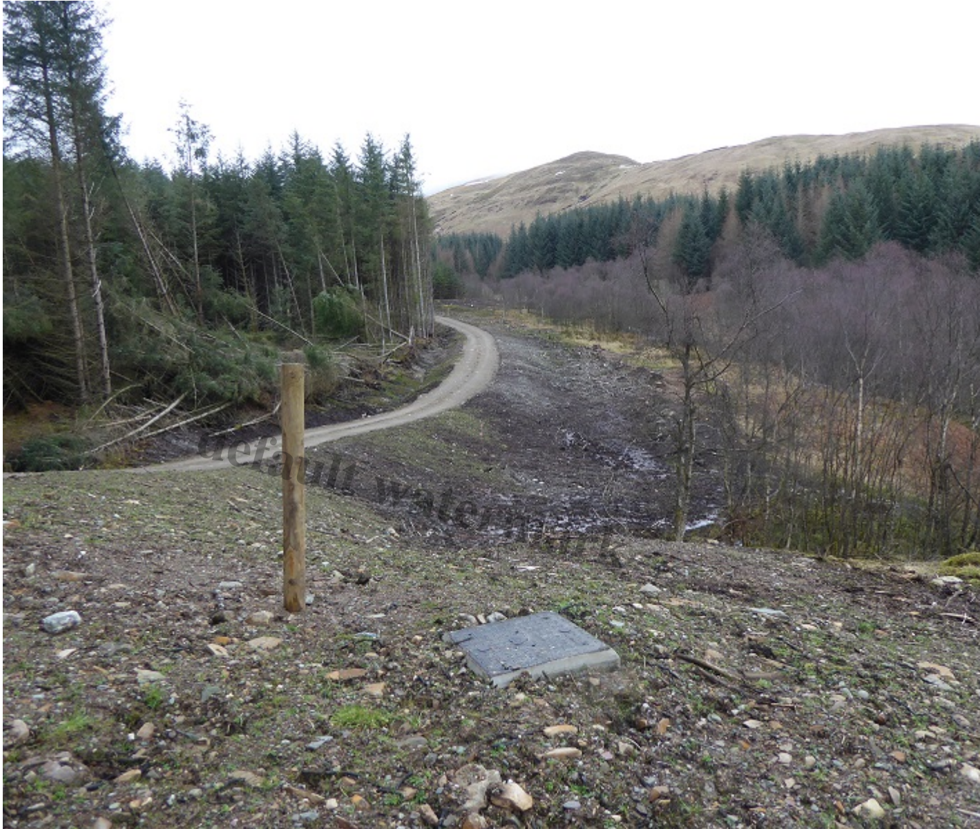
Looking up the track and pipeline towards Ben Ledi
