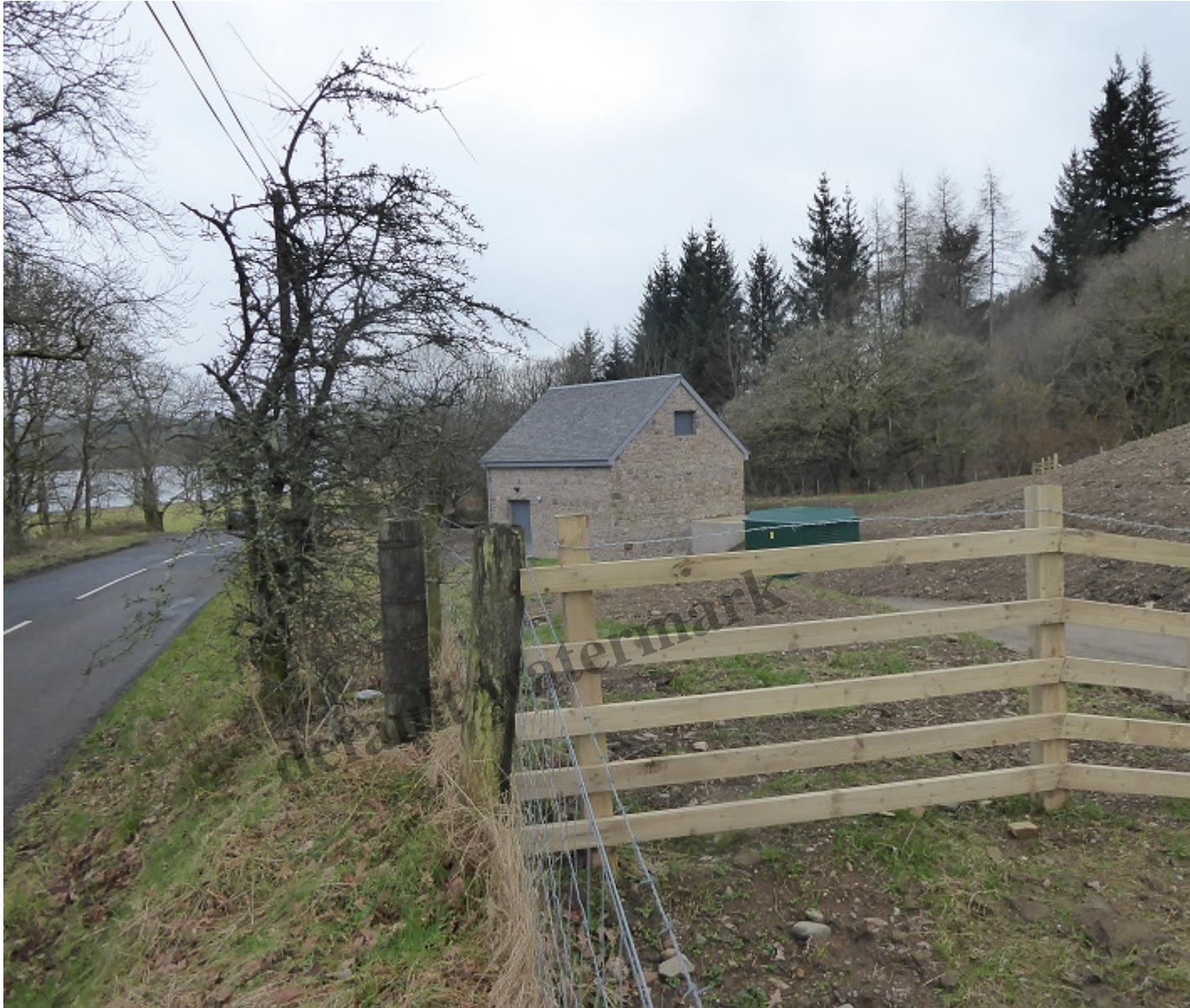
Milton Glen powerhouse viewed in 2016
