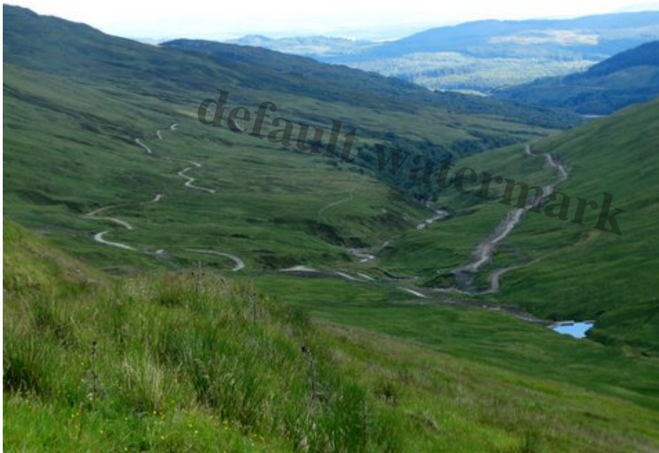
Gleann Casaig Hydro Oct 2017, the original track which was extended to the intake (the pool) on the left, the new track to the right. Photo Credit Jim Robertson
