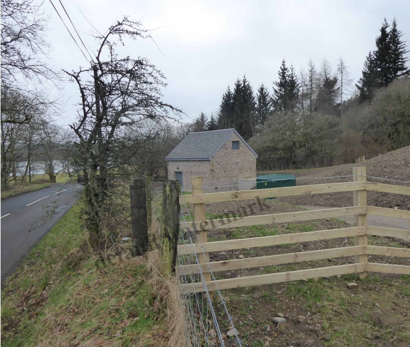
Milton Glen powerhouse viewed in 2016
