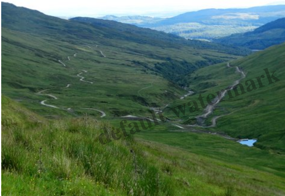
Gleann Casaig Hydro Oct 2017, the original track which was extended to the intake (the pool) on the left, the new track to the right. Photo Credit Jim Robertson
