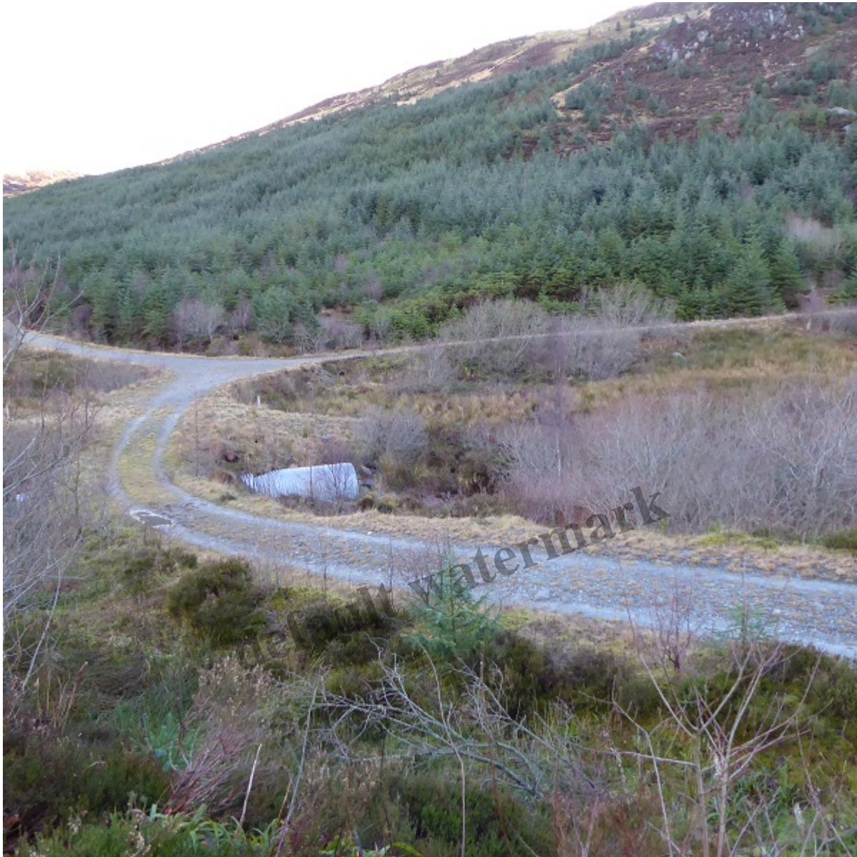
Forestry culvert under the track just below the intake – the hydro pipe lies under the line of rush just behind.
