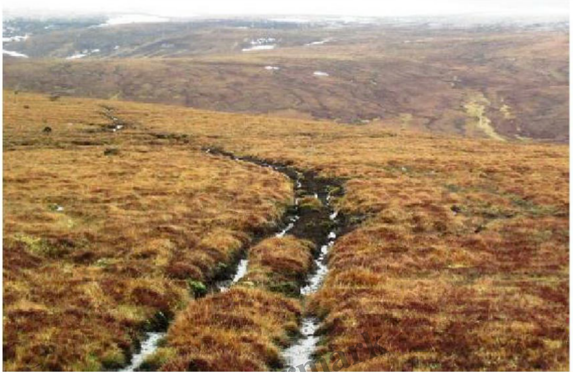
Plate 7. Existing track cuts through the blanket bog towards the River Dulnain. Peat depths were consistently 1 m on average either side of the track here.
