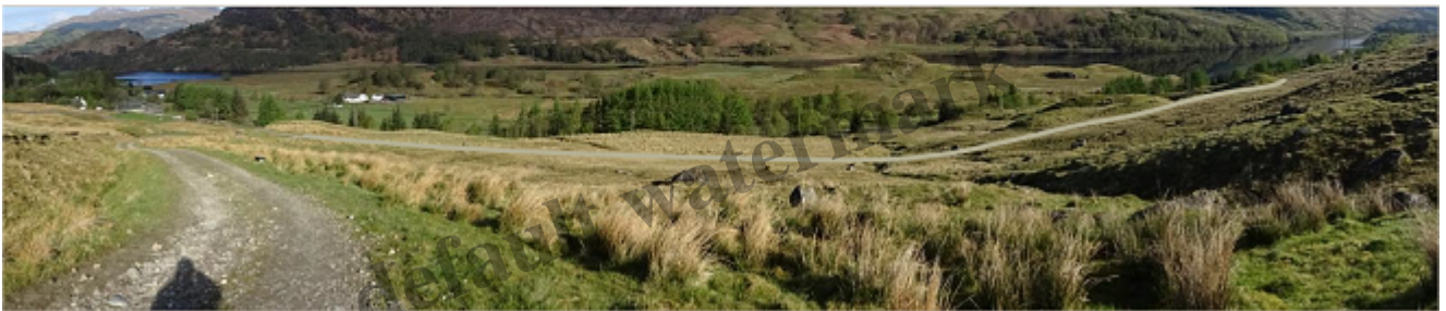
View of the power house connecting track from above: top – current view; middle – line of route; bottom – photomontage
