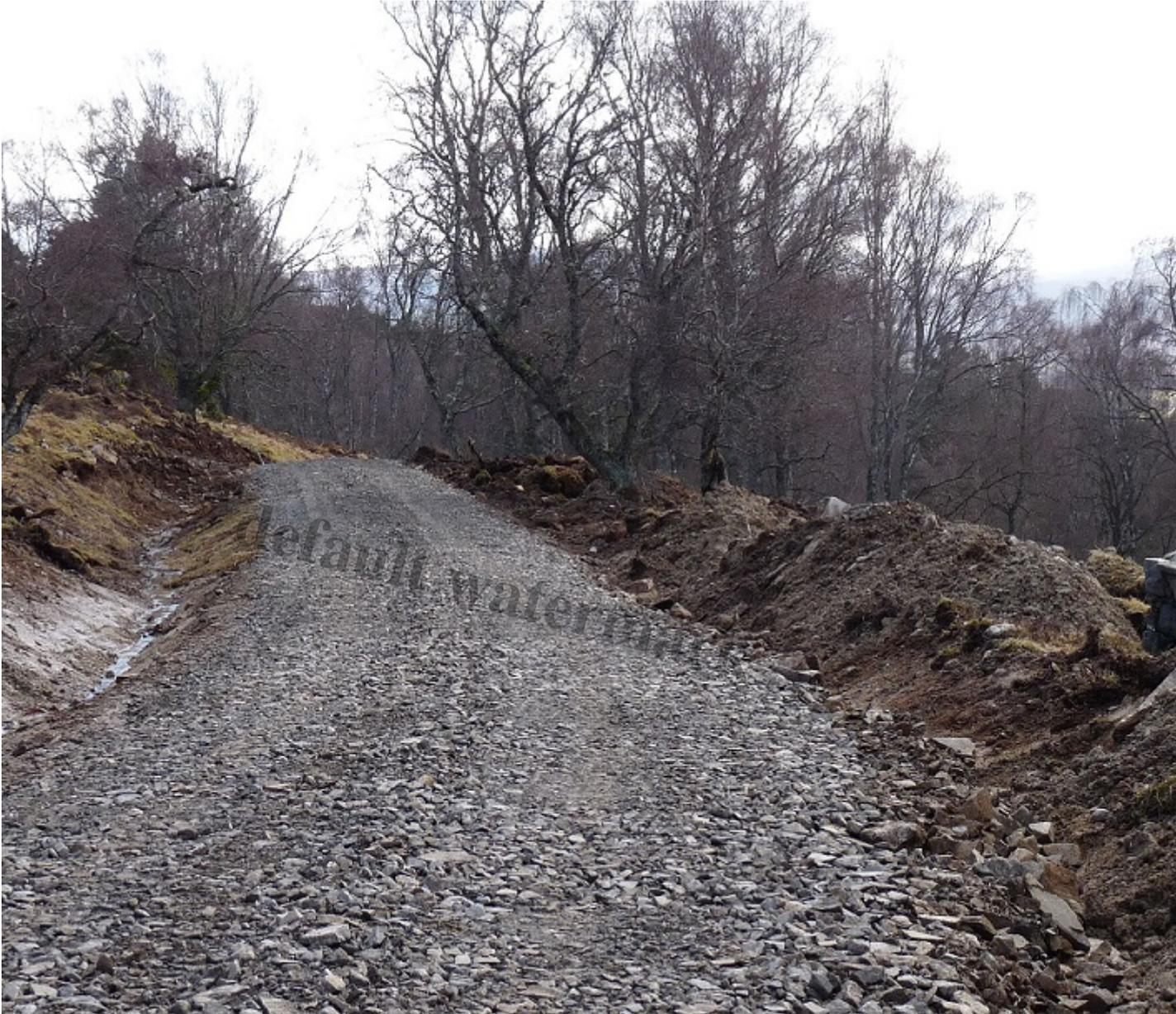
Upgrading work in progress showing the extent of the ground affected and the width of the track
