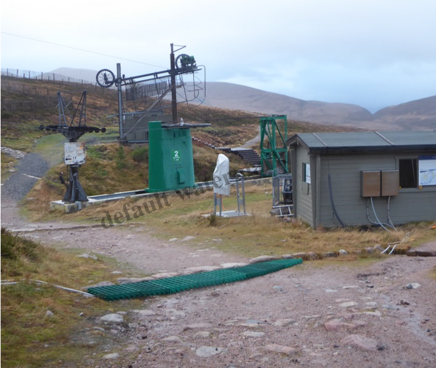
New wiring for snow cannon opposite the Day Lodge – Photo Nick Kempe
