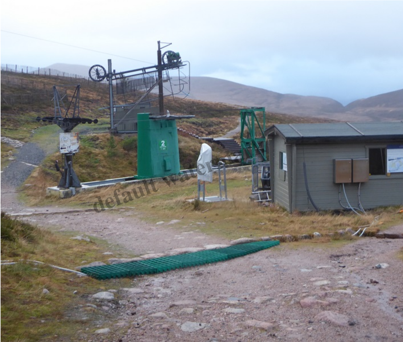
New wiring for snow cannon opposite the Day Lodge – Photo Nick Kempe
