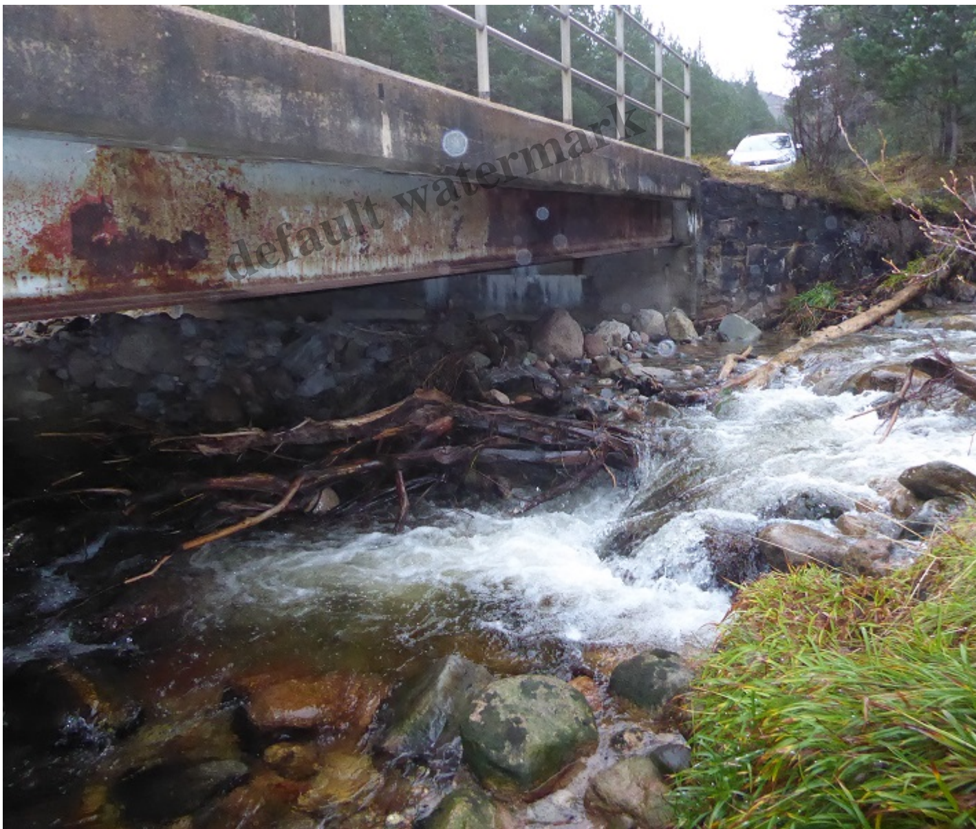
The bridge over the Allt Mhor near the bottom of the ski road 24th November 2018, half-blocked by t
