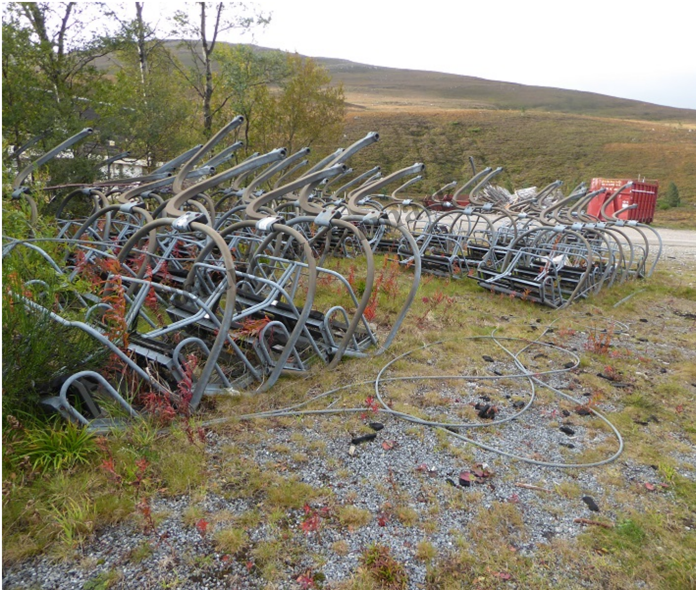
Coire na Ciste is still like a builders' yard despite the clear up last year paid for by HIE
