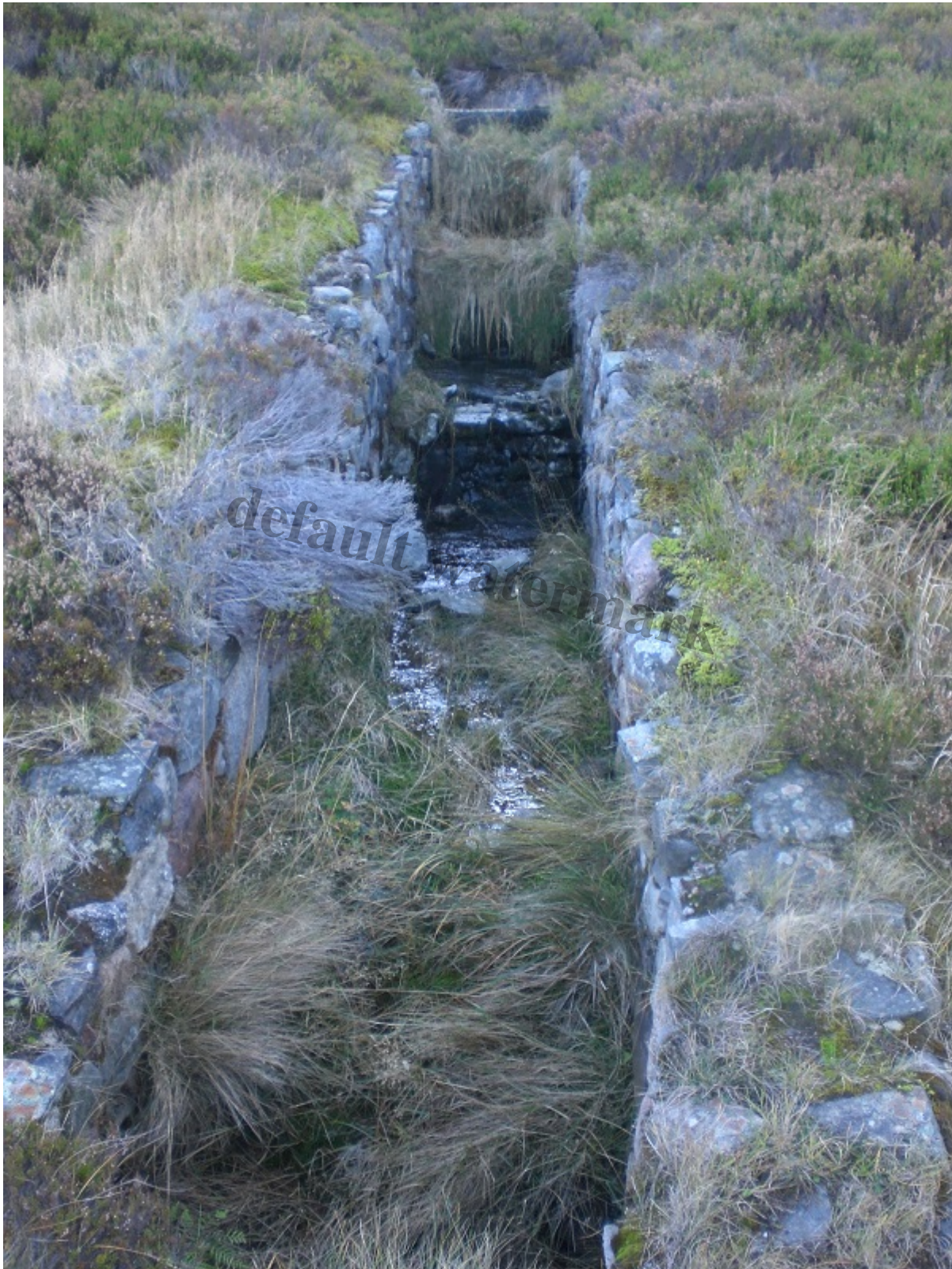
Drainage channel above link road Nov 2018 Photo Credit Alan Bratney
