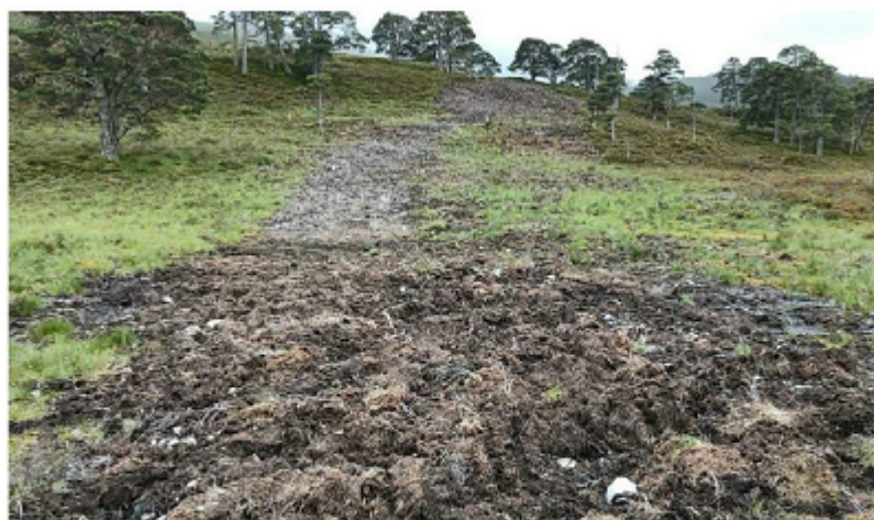
Figure 3.8 A restored pipe trench, this one in the Glen Affric National Scenic Area and Strathglass Complex SAC, shortly after it was backfilled and the surface restored. Once vegetation is established on the bare peat the pipe route will be completely invisible.
