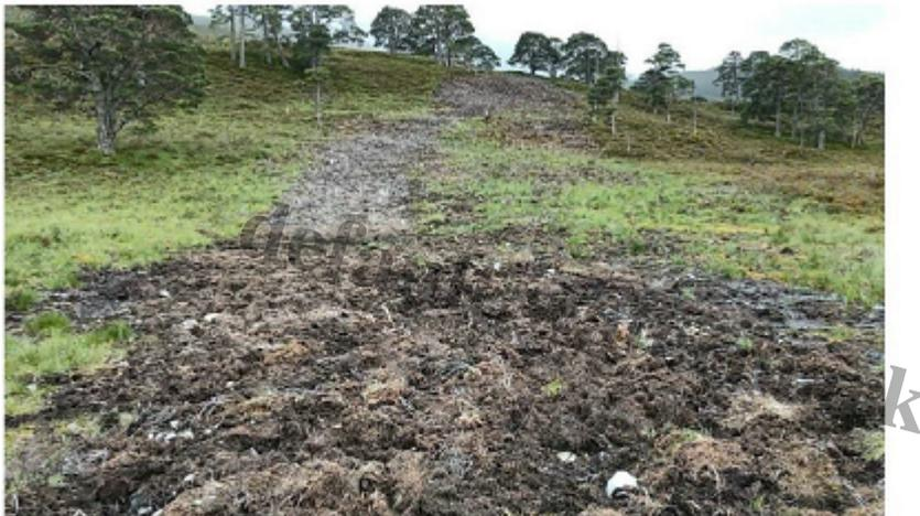
**Figure 3.8 A restored pipe trench, this one in the Glen Affric National Scenic Area and Strathglass Complex SAC, shortly after it was backfilled and the surface restored. Once vegetation is established on the bare peat the pipe route will be completely invisible.**
