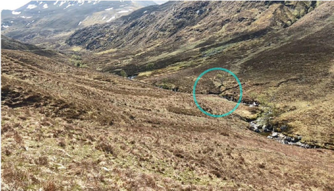
Figure 3.26 Looking towards the west intake (circled) on the Allt Leachdach, Scheme 5. The Lairig Leacach track can be seen contouring along the side of the glen on the left of the picture.
