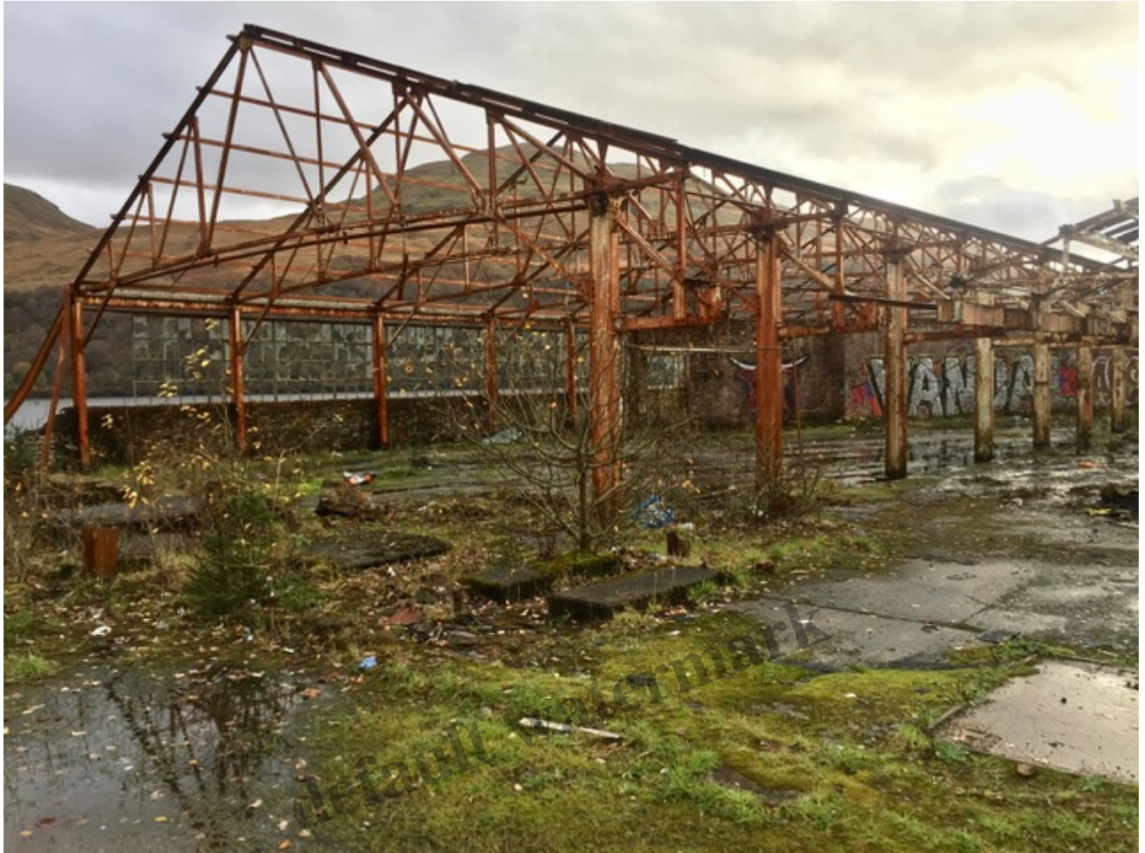
Halted demolition – Photo Credit Nick Halls
