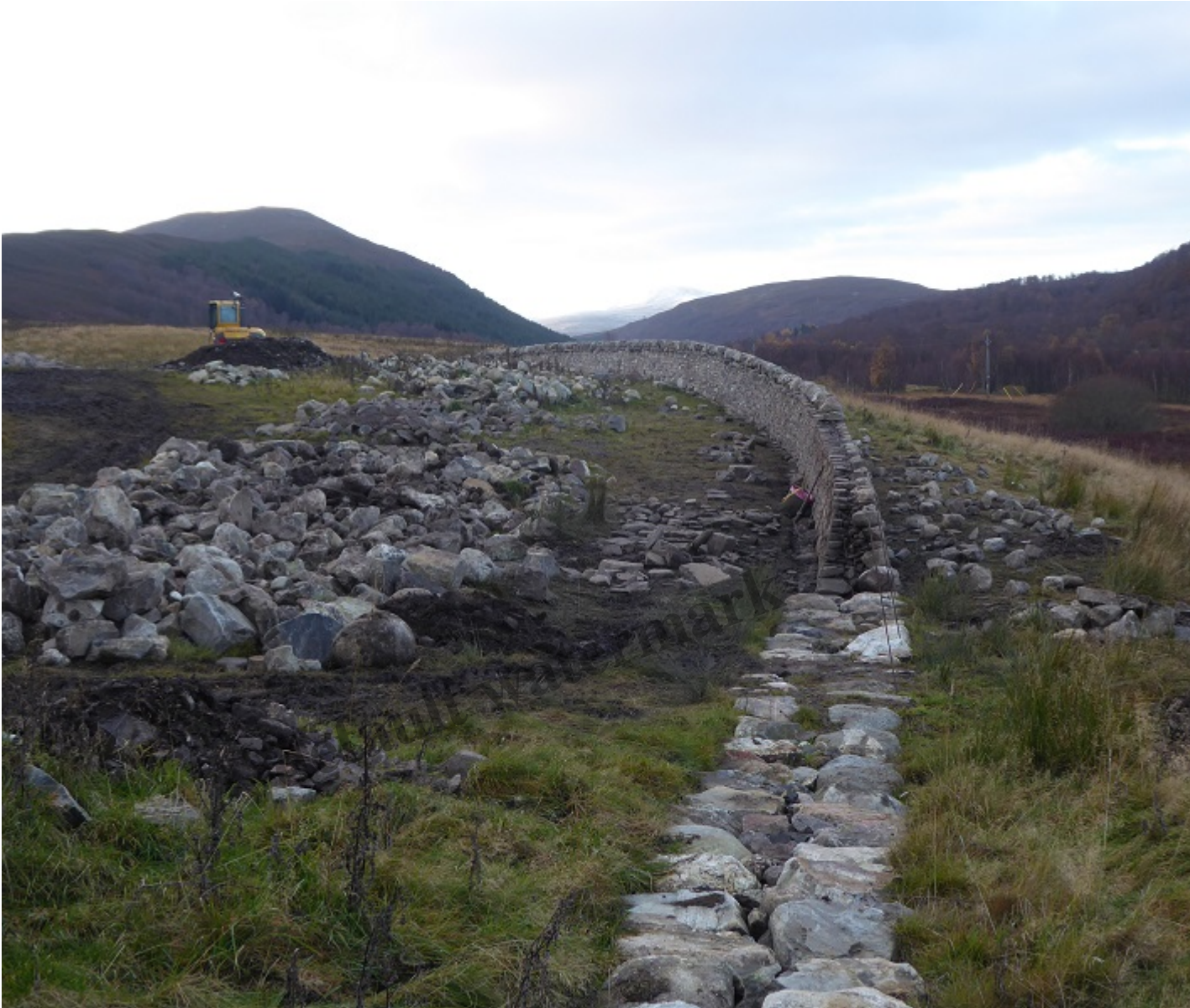
Dry stane wall building in Glen Tromie by Killiehuntly Oct 2017 – such landscaping work supports local employment
