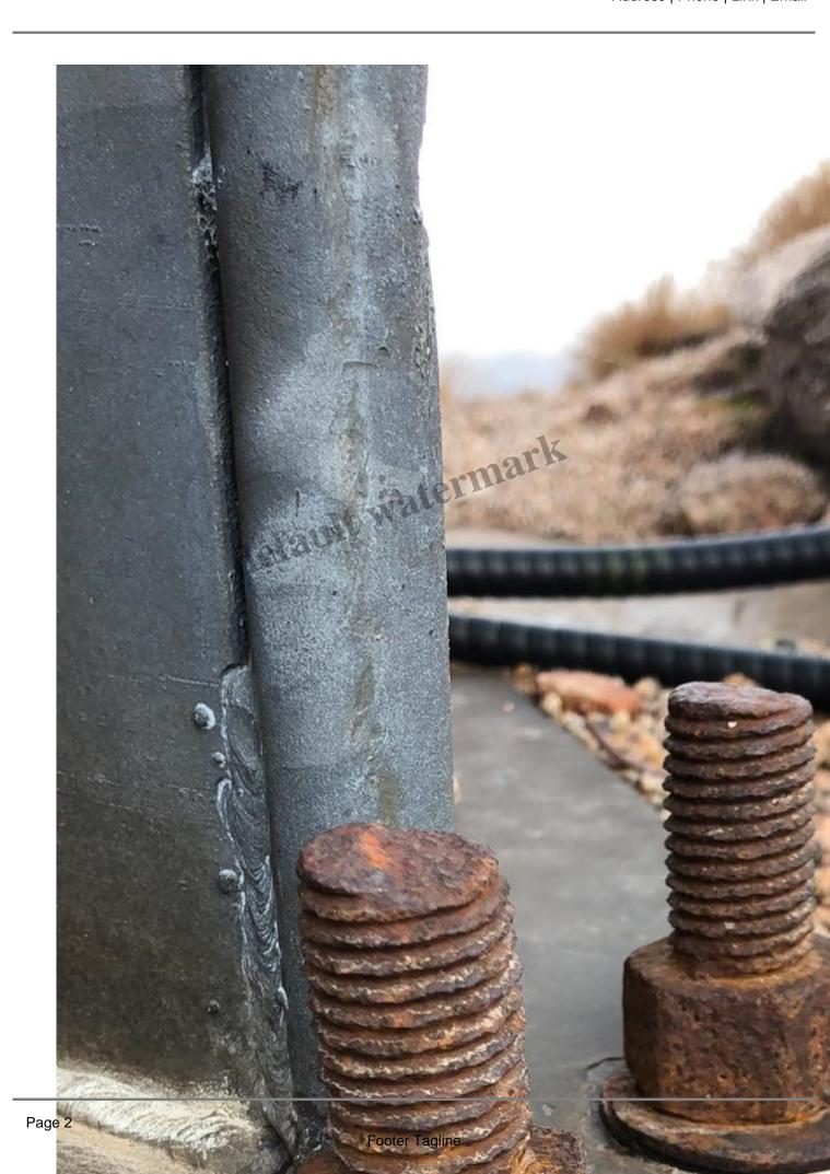
Rusted and corroded bolts Ptarmigan t-bar – recommendations to fix these in 2015, 2016 and 2017 Brattey
