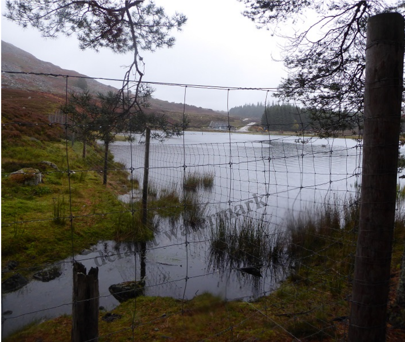
The view from the north east corner of the plantation from close to the fence looking over to the Gyn powerhouse on far side of bay (centre)
