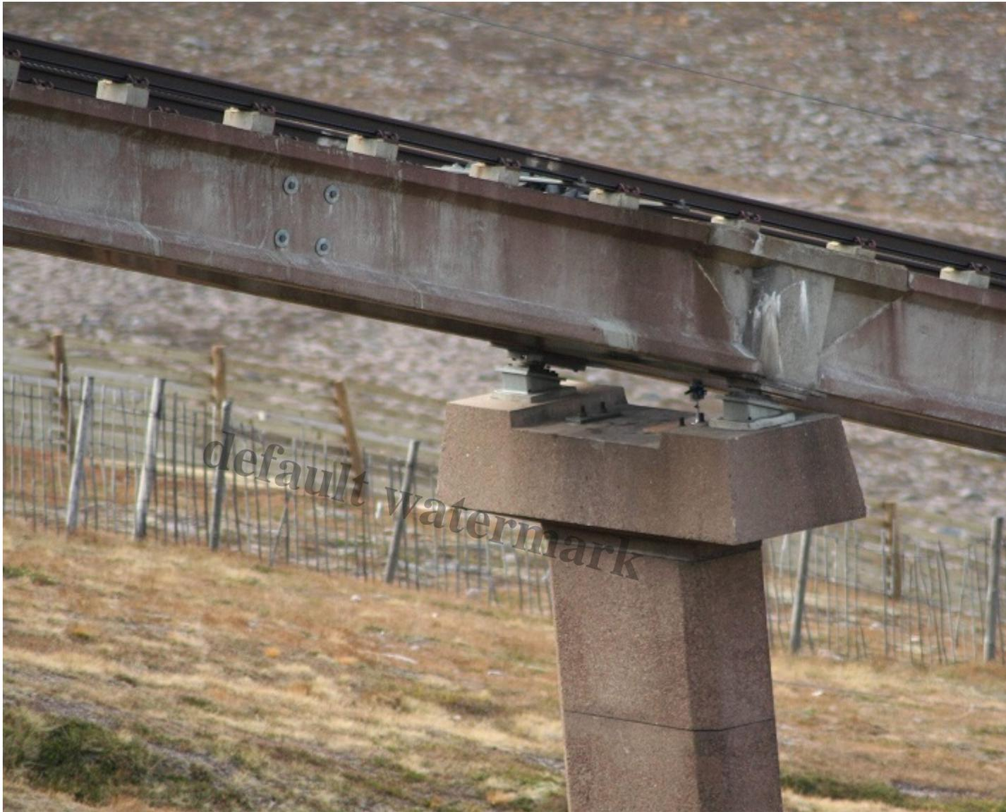
Monitoring device at tunnel mouth – note the apparent cracks in the t-section above. Photo credit
