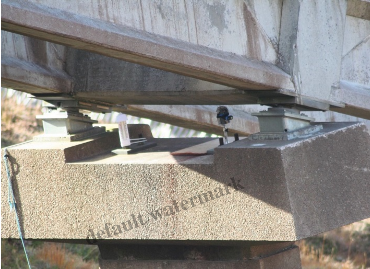
Monitoring device and thermometer just above the mid-station. Photo credit Terry Smith
