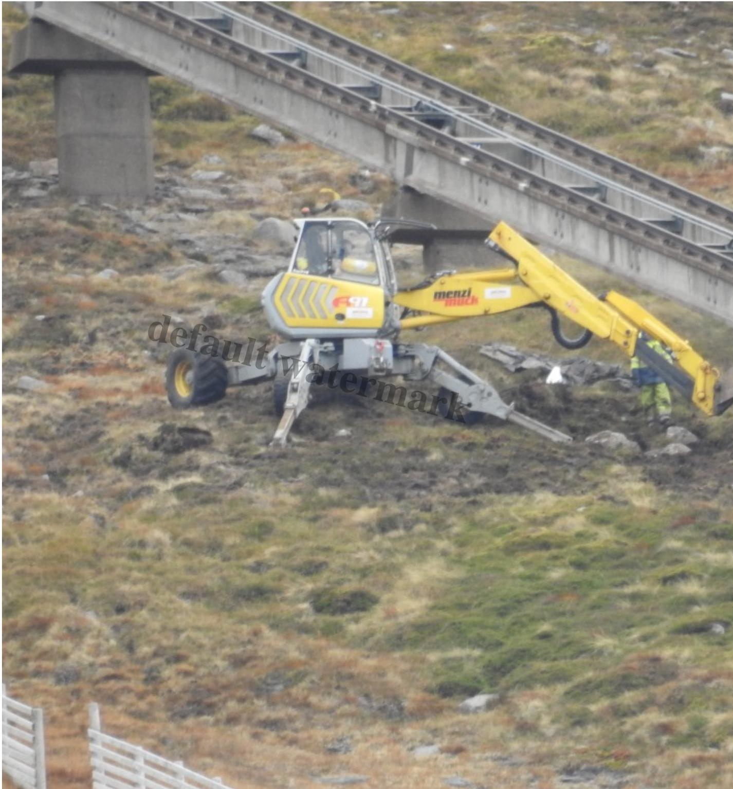
Digger excavating one of the shoogly pillars 18th October (apparently the pillar below the one in the measures being taken to protect the ground. Photo Credit Gus Jones
