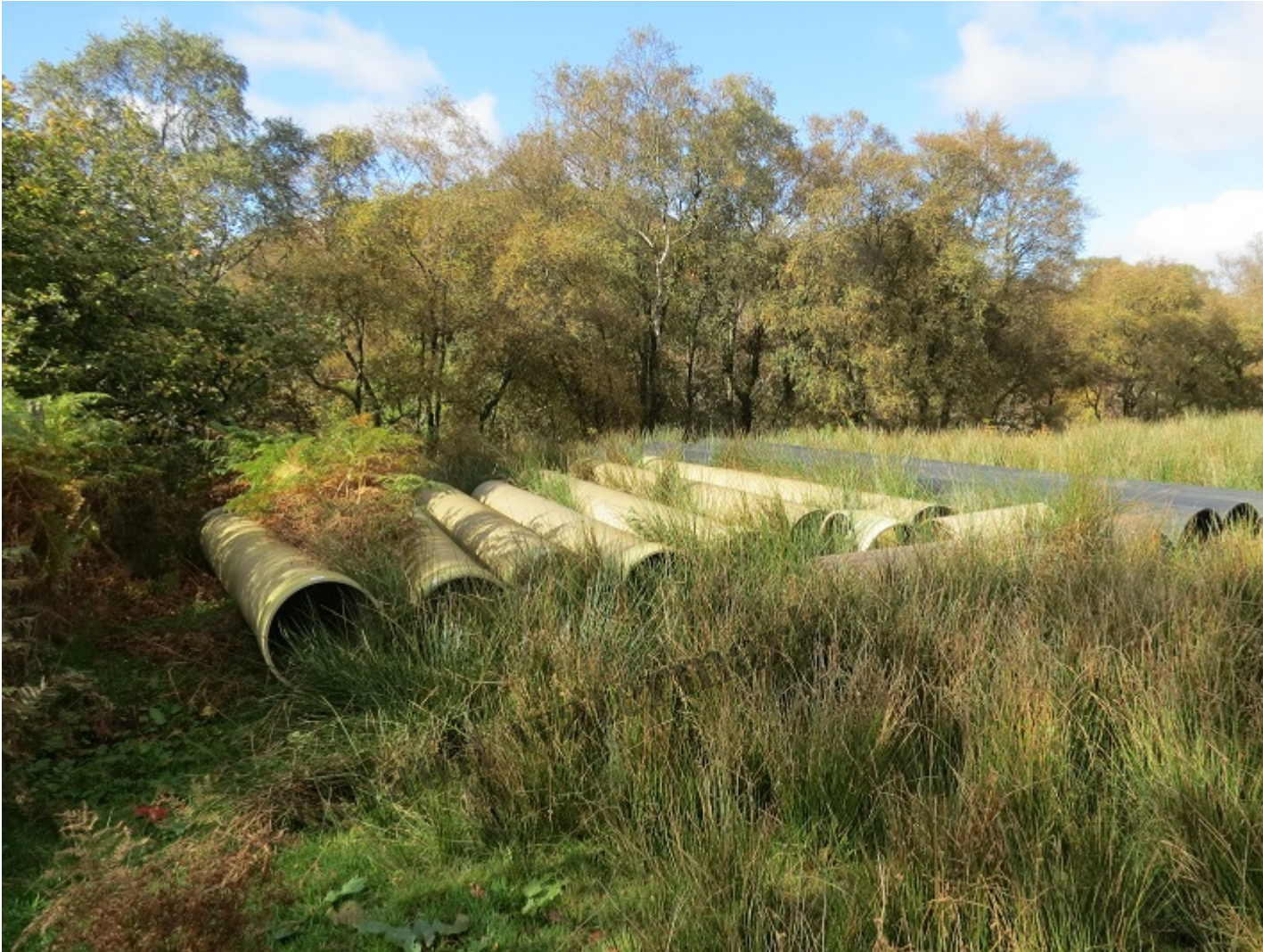
Two types of hydro pipes, glass reinforced plastic for use lower down where the water pressure is high and the black for use higher up. Photo credit Louise Brimelow.
