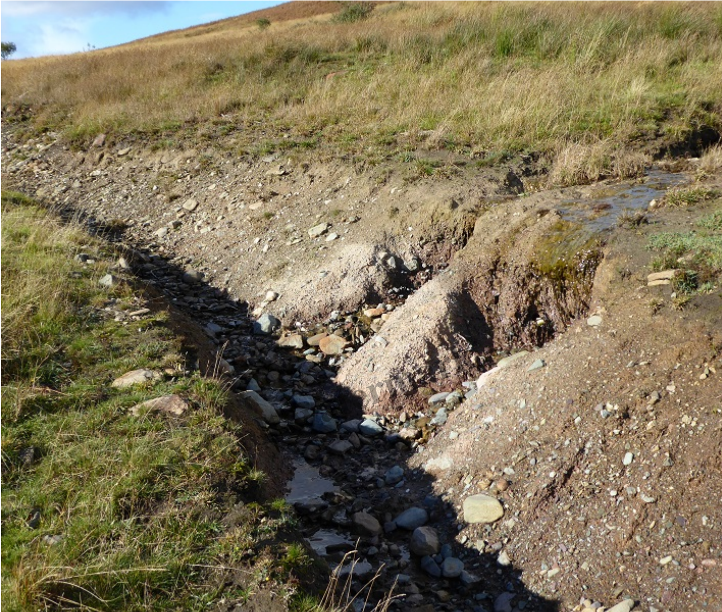
Unrestored drainage ditch showing impact of water erosion running down the bare sides from above
