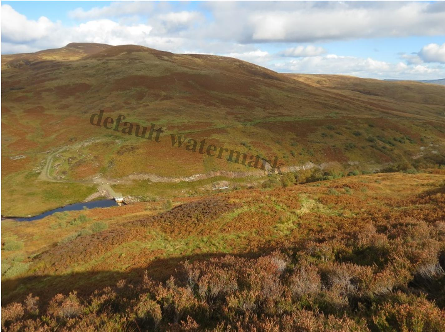
The upper section of the Burn of Mar hydro scheme from from Conic Hill showing the intake, the new track curving up and back across the hill and the scar left by the construction of the pipeline. Maol O Photo Credit Louise Brimelow.
