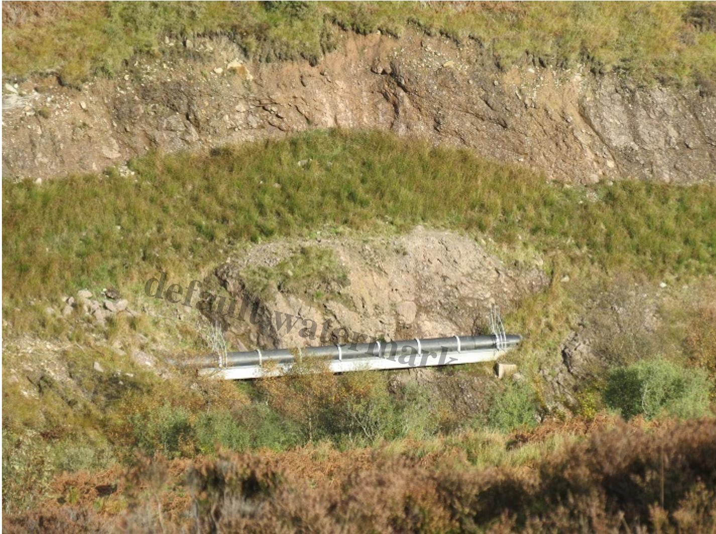
Close up of pipe bridge below two areas of excavated hillside. The line of rush between the two marks the "restored" construction track. The construction corridor here was supposed to be a maximum wide
