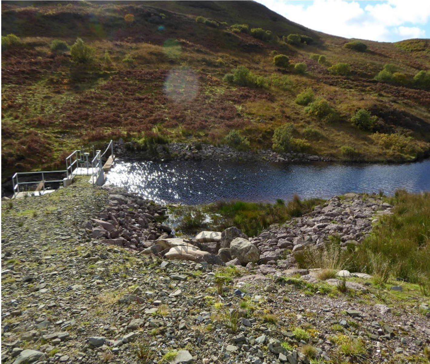
View in opposite direction back to intake
