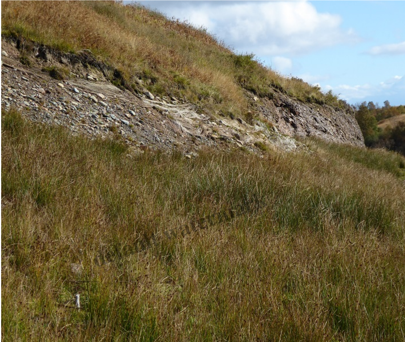
The landscape scar viewed from round the corner closer to the intake
