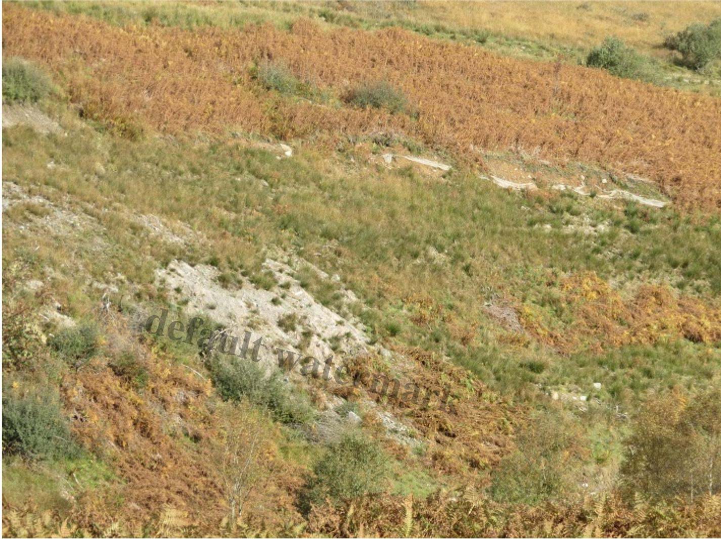
Same view, through telephoto lens. Note the textile matter across the bare earth slope and the spoil appears to have been dumped below the line of the pipe. Photo Credit Louise Brimelow.
