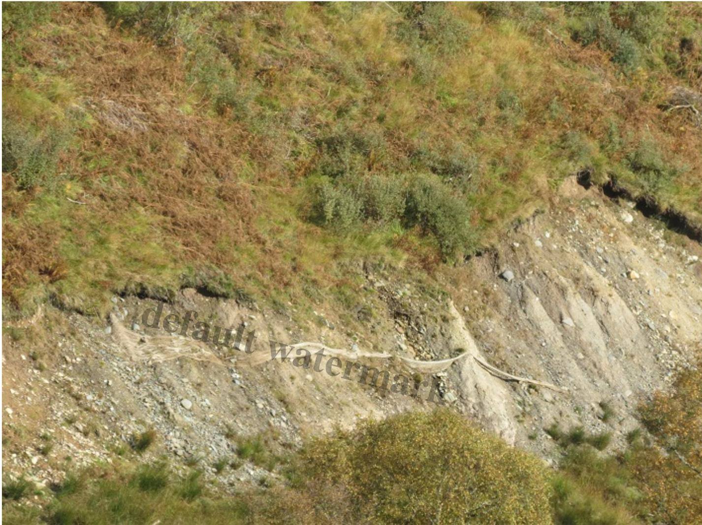
Same section more or less viewed from different angle. Note how the textile matting has clearly failed and water has eroded the exposed slope to the right of this
