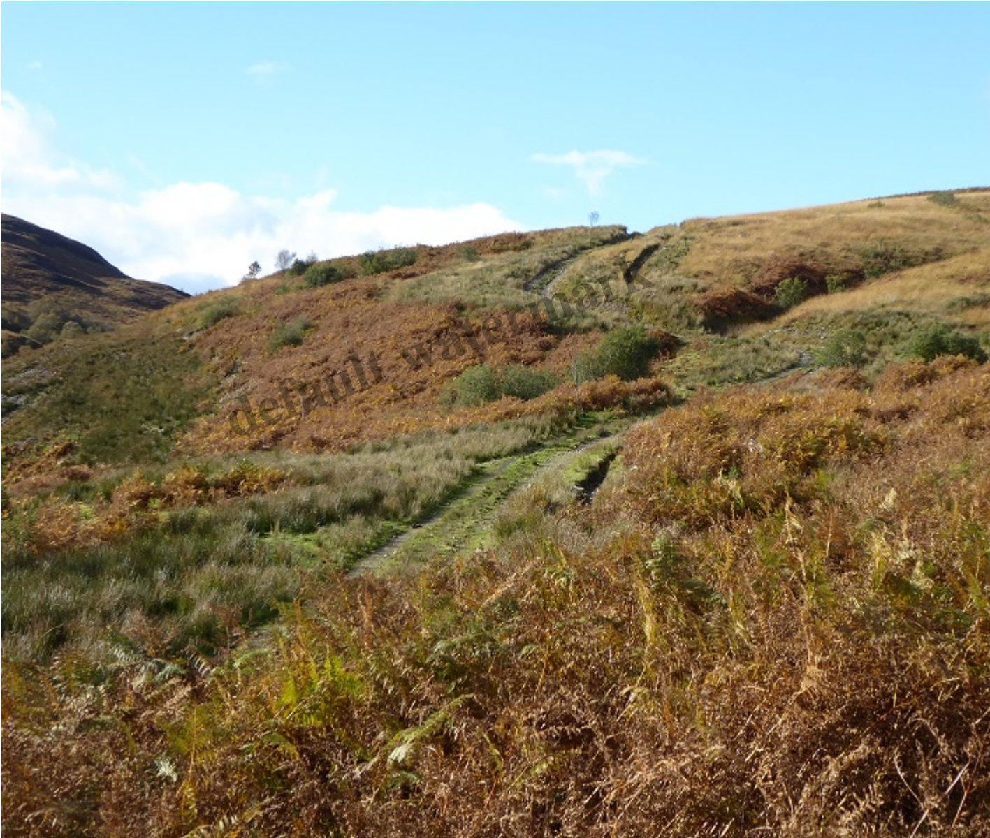
The new track from just above where it crosses the West Highland Way – note how the enormous ditch on the right has almost as much impact as the track itself.
