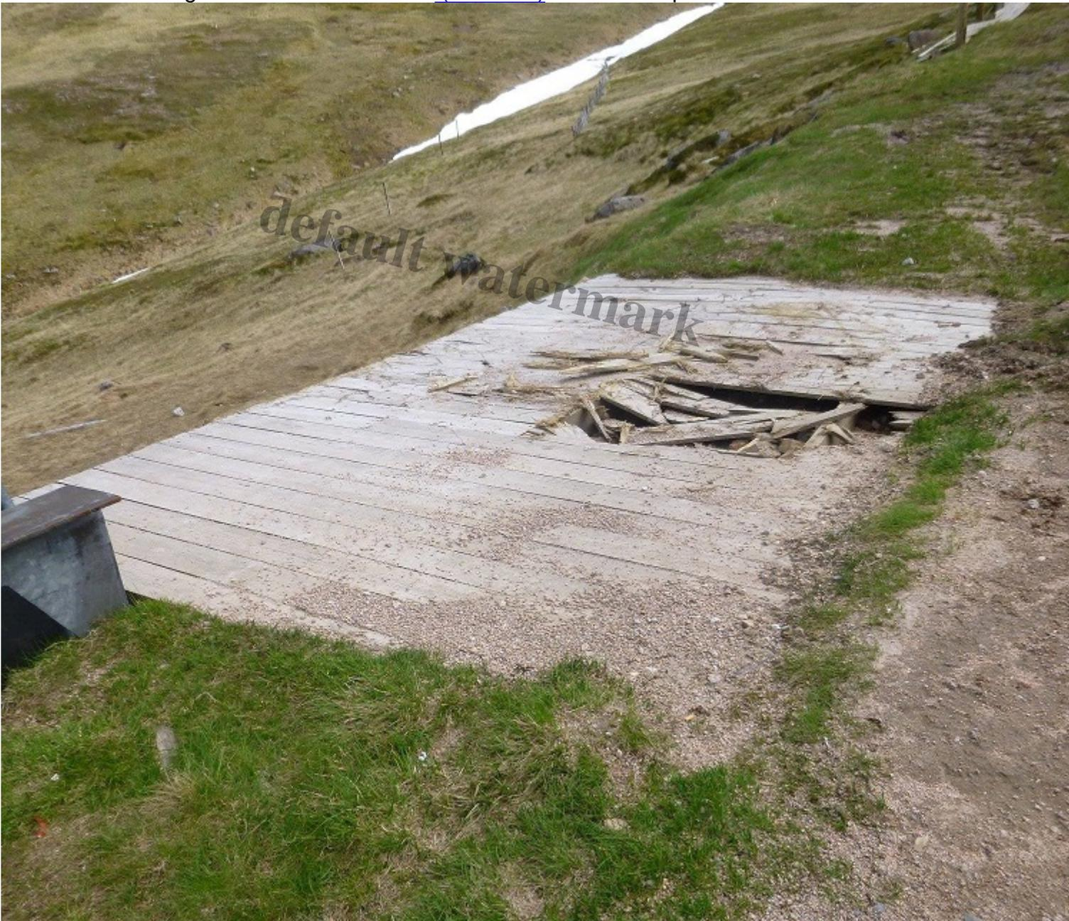
This was highlighted in the ADAC structures report in 2015 *“A review of the access platform is recommended”* and the again in the 2016 report *“The timber platform was seen to be broken, possibly due to vehicle access – this needs to be replaced before the coming season. This was discussed with CML (Cairngorm Mountain Ltd) staff at the time and assurance that this would be*
