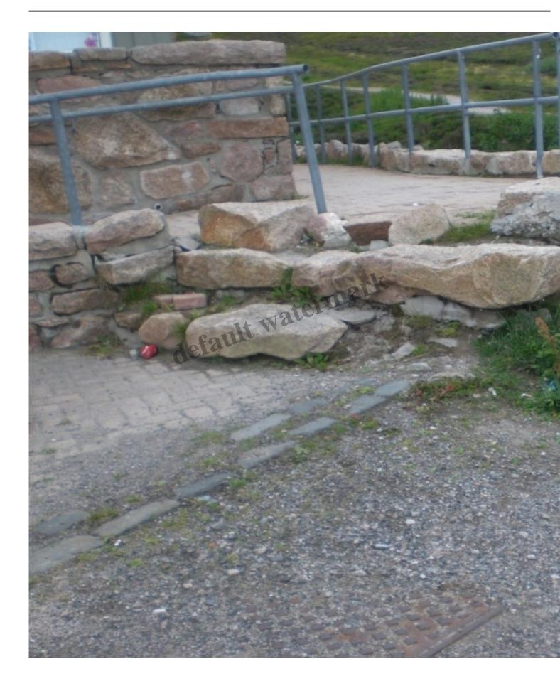
This picture is of the area at the corner of the Daylodge closest to the CarPark T-Bar. There has been no maintenance done here for several years and it is clearly in a state of collapse. A large granite block has fallen out of the wall which could have seriously injured any child who had been climbing on it, as children do.
