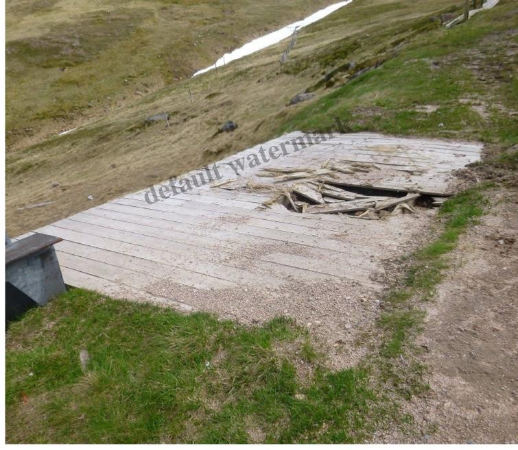
This was highlighted in the ADAC structures report in 2015 'A review of the access platform is recommended" and the again in the 2016 report "The timber platform was seen to be broken, possibly due to vehicle access – this needs to be replaced before the coming season. This was discussed with CML (Cairngorm Mountain Ltd) staff at the time and assurance that this would be done were received".
