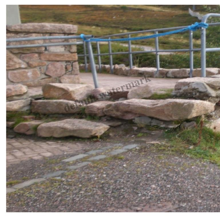
Someone clearly thought that tying on a piece of rope where there should be a barrier, would do the job!
