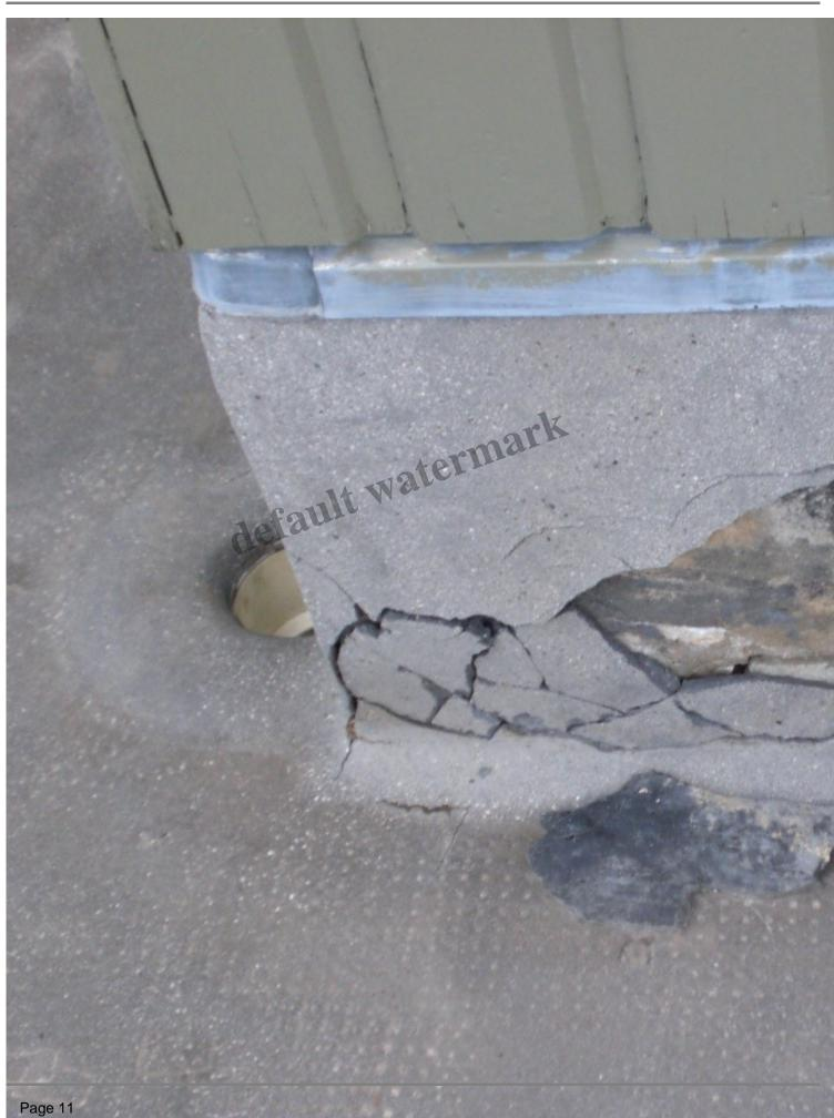
.....the flashing on the walk ways is in a state of disintegration.
