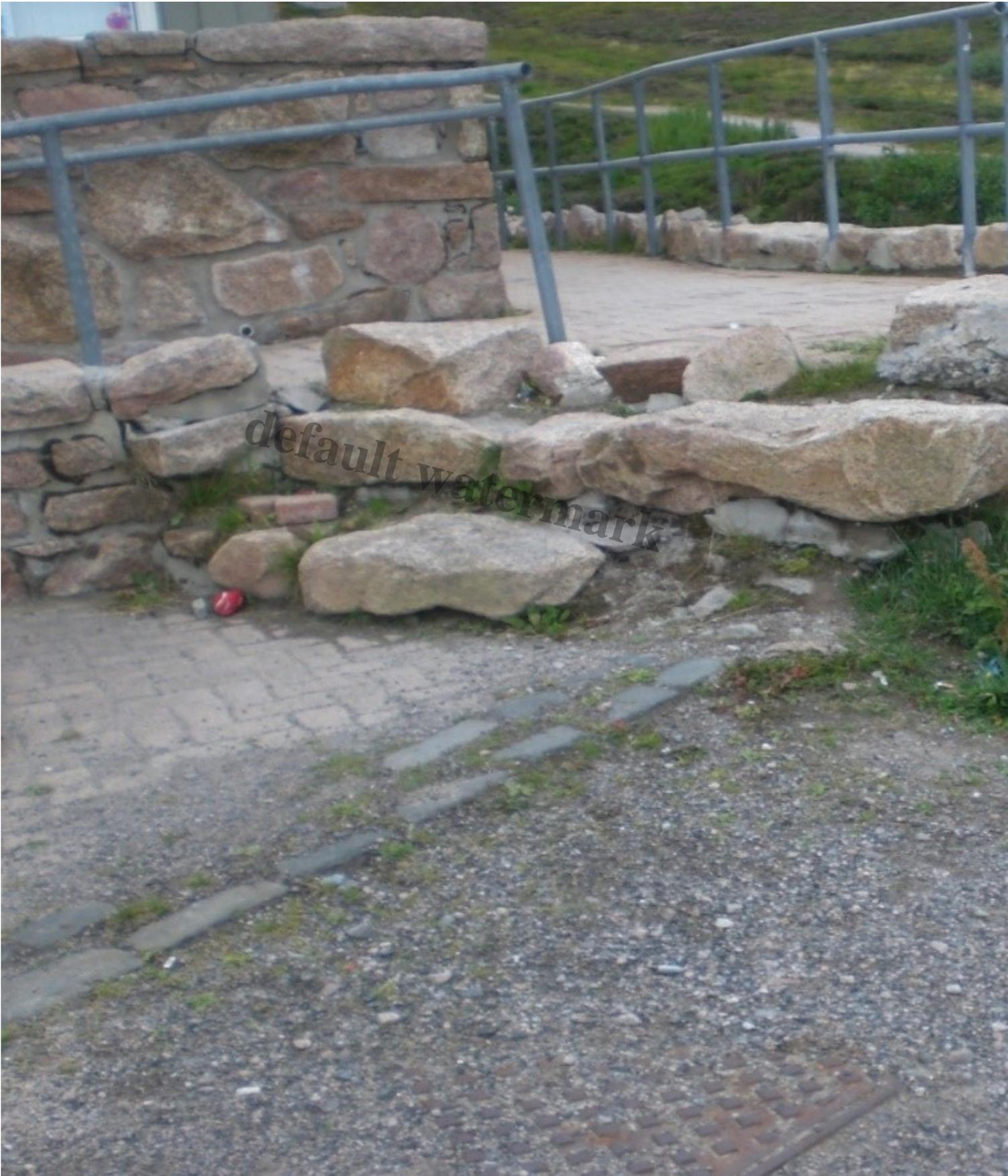
This picture is of the area at the corner of the Daylodge closest to the CarPark T-Bar. There has been no maintenance done here for several years and it is clearly in a state of collapse. A large granite block has fallen out of the wall which could have seriously injured any child who had been climbing on it, as children do.
