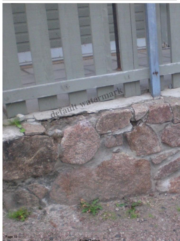
.....yet more collapsing granite walls with no sign of anything having been done by way of repair or maintenance for some years
