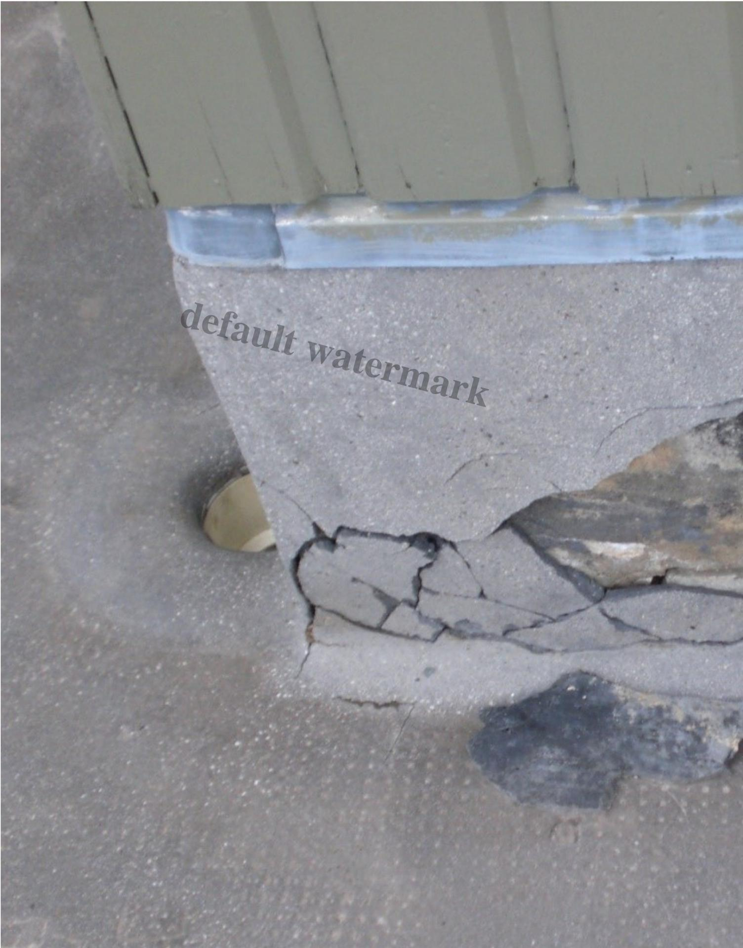
the flashing on the walk ways is in a state of disintegration.
