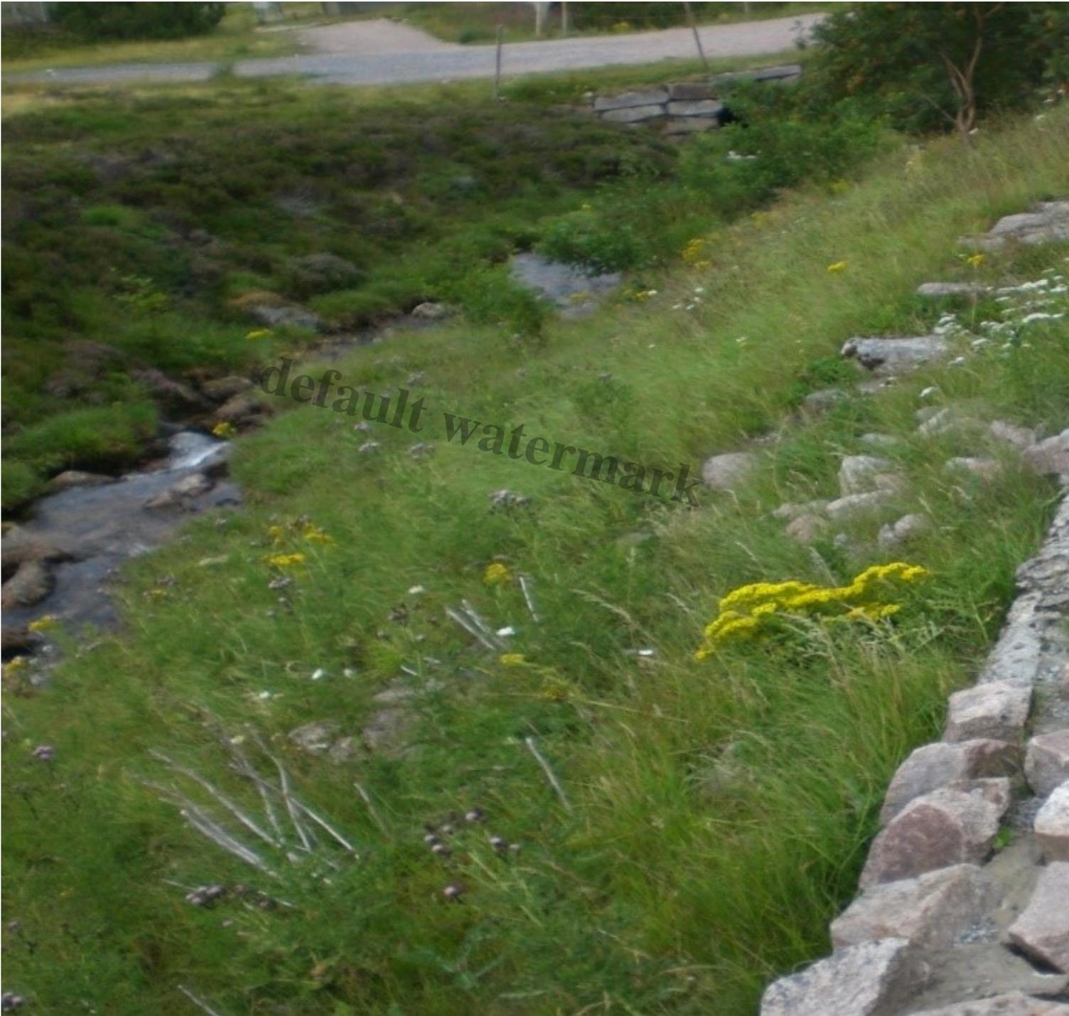
The dwarf wall has more or less completely collapsed and fallen down the slope towards the burn.
