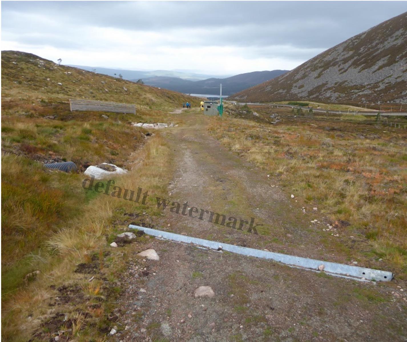
Looking down the bottom section of the Shieling track, note the protruding plastic culvert on left
