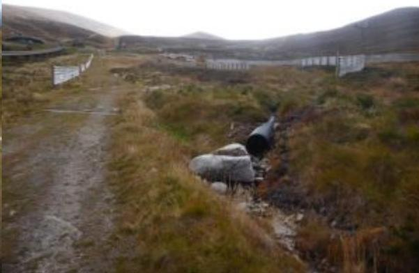
The original planning application for the Sheiling tow referred to new culverts to channel the Allt Choire Chais, which the Construction Method Statement stated would be carefully covered over, but nothing about these culverts or the other plastic culverts that have inserted in other areas outwith the area granted planning permission:
