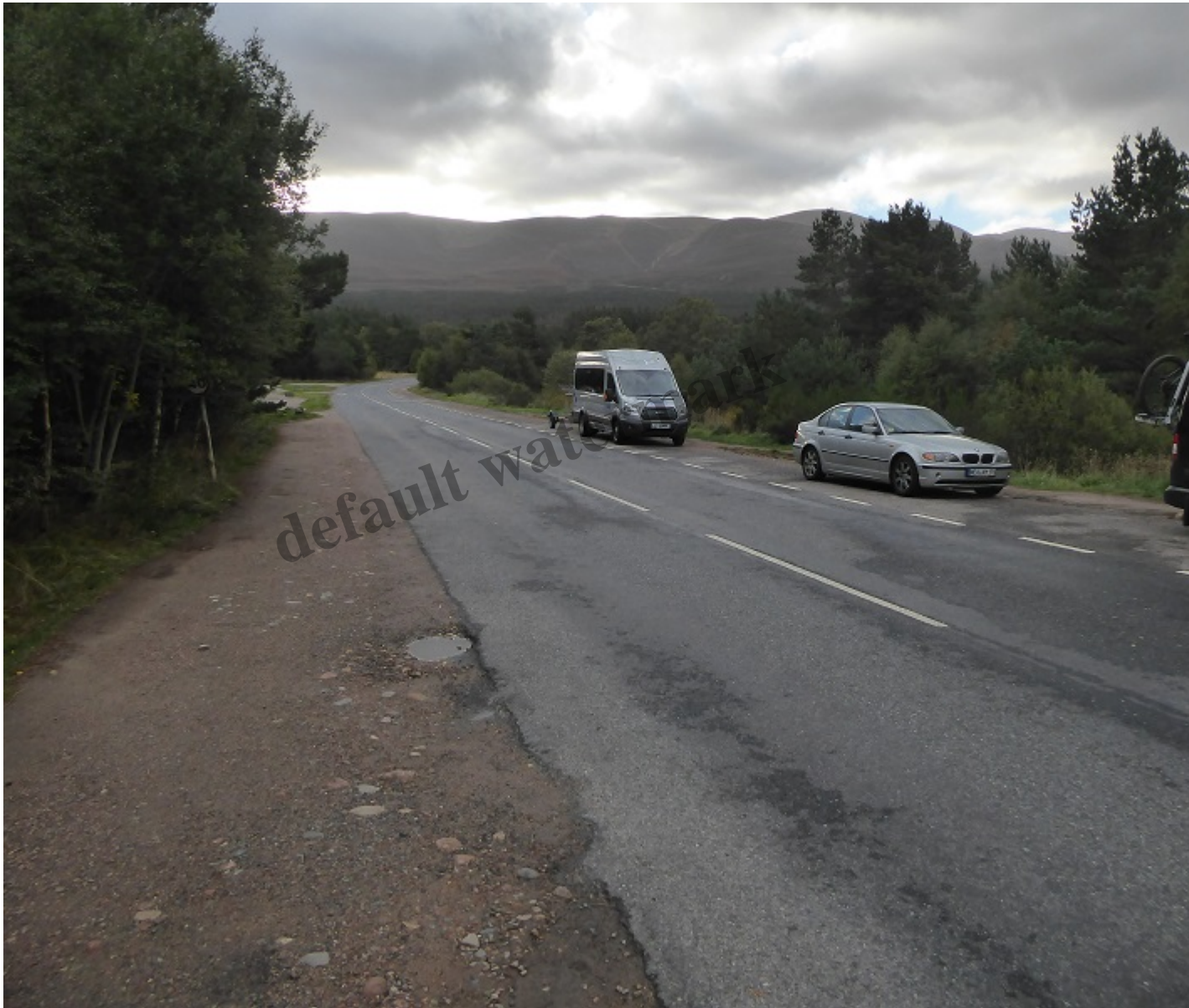
Looking towards the Hayfield earlier this week – the parked cars make it difficult for people to walk alongside this section of road
