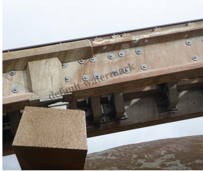
Crack in horizontal beam (below rail) just above funicular mid-station. You can see further signs of c between bolts below
