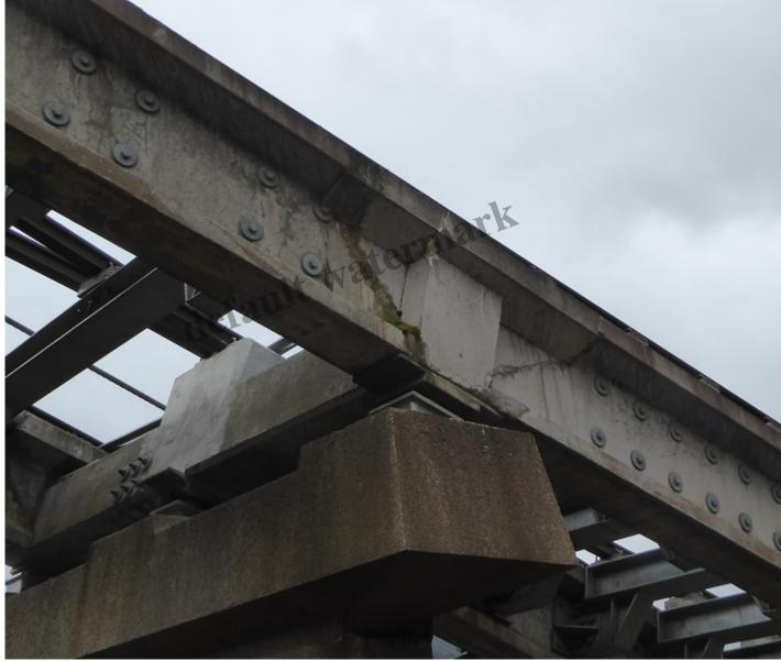
These cracks were on either side of a support column where the railway splits to allow carriages to p
