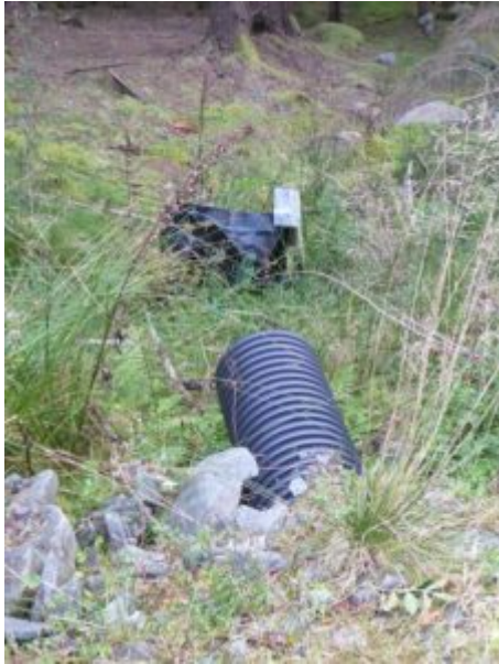
Protruding culvert on new section access track
