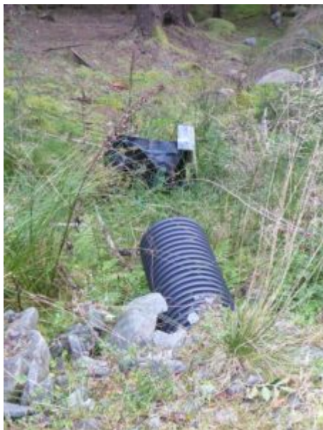
Protruding culvert on new section access track
