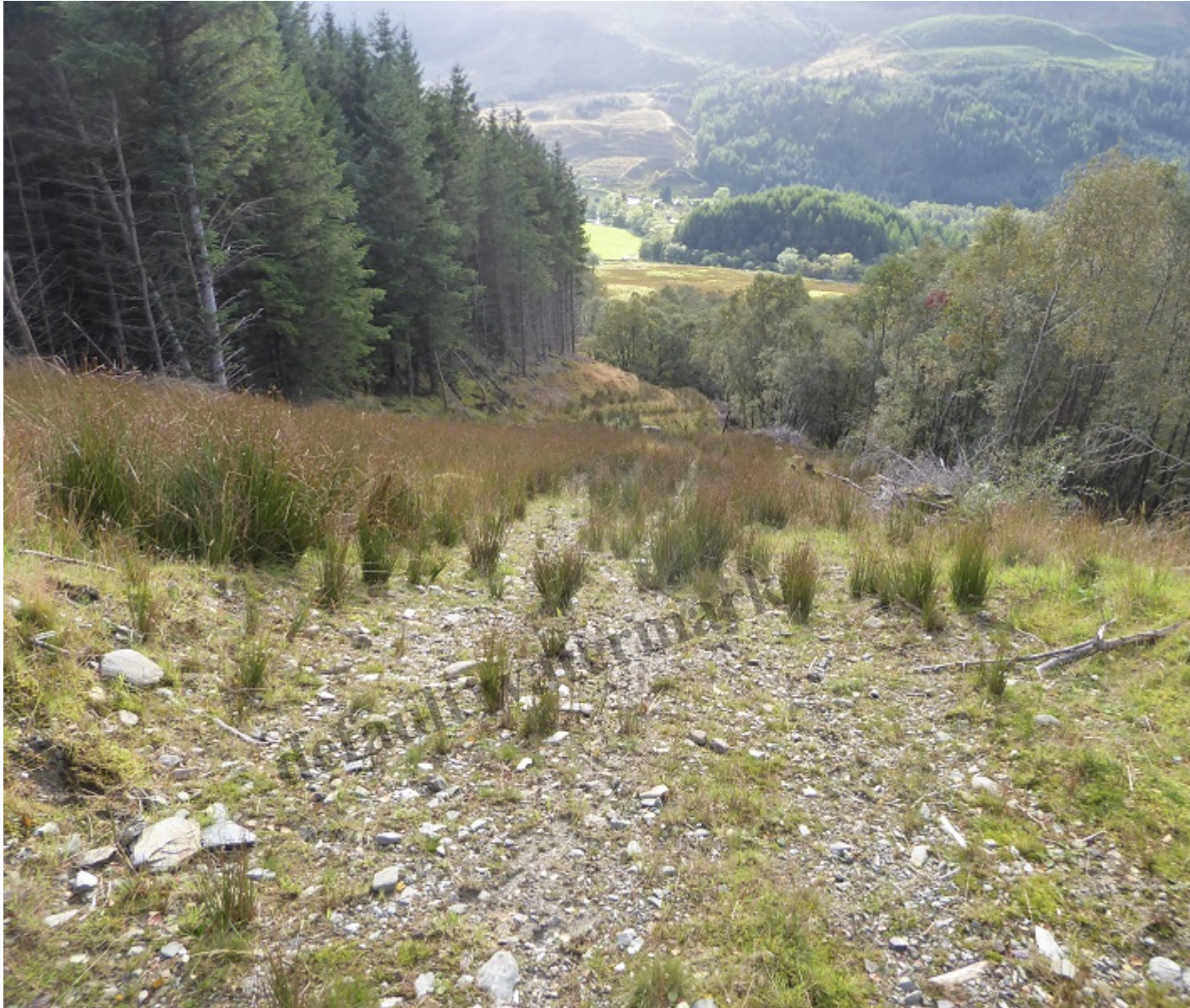
More restoration failure of the pipeline below the forest track
