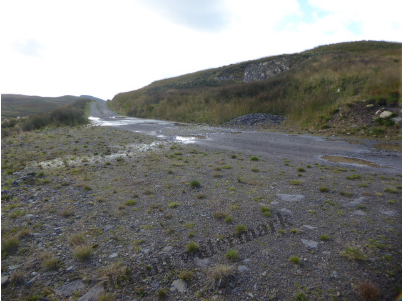
Unrestored ground with heap of aggregate behind and only partially restored borrow pit behind.
