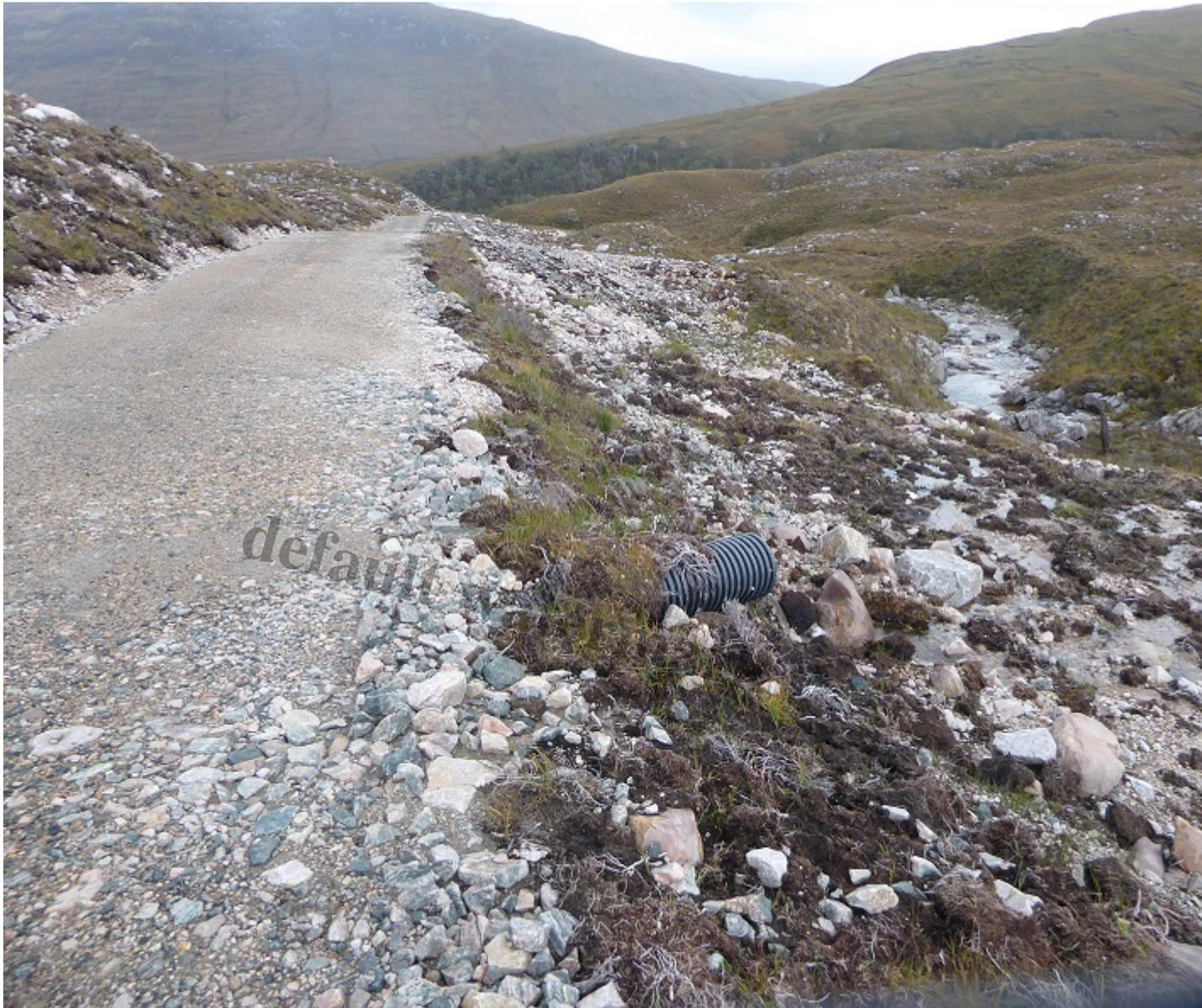
Lower down vegetation has been replaced either side of the track even if the ground below the track is messed up with soils and vegetation mixed contrary to the Construction Method Statement. How plastic culverts are compatible with the protection of National Scenic and Wild Land areas is unclear.
