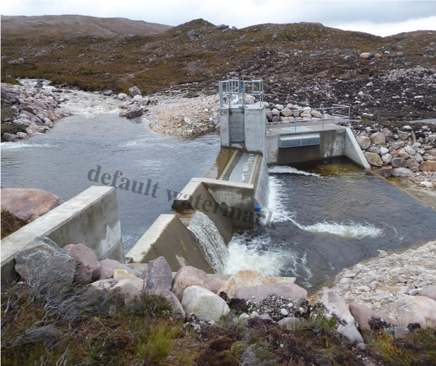
The extensive use of rip rap bouldering to reduce erosion of the rivers above and below the intake w long-term landscape scar â?? vegetation is unlikely to be able to colonise such bouldering for a very
