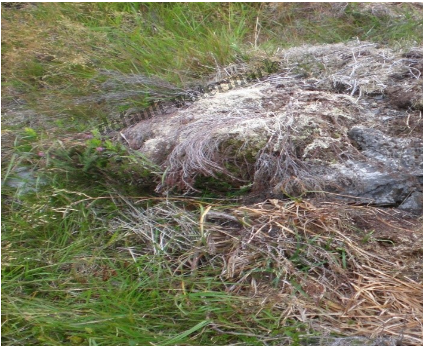
Exposed concrete which has not been broken out to 200mm below surface. Photo Credit Alan Bratt
