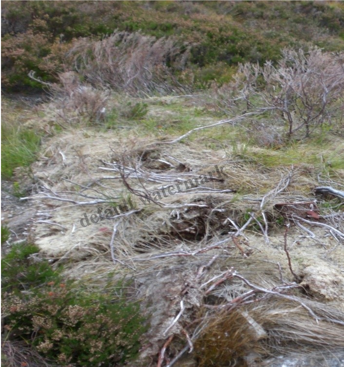
Concrete coverage: Note how the vegetation has died. Photo Credit Alan Bratney
