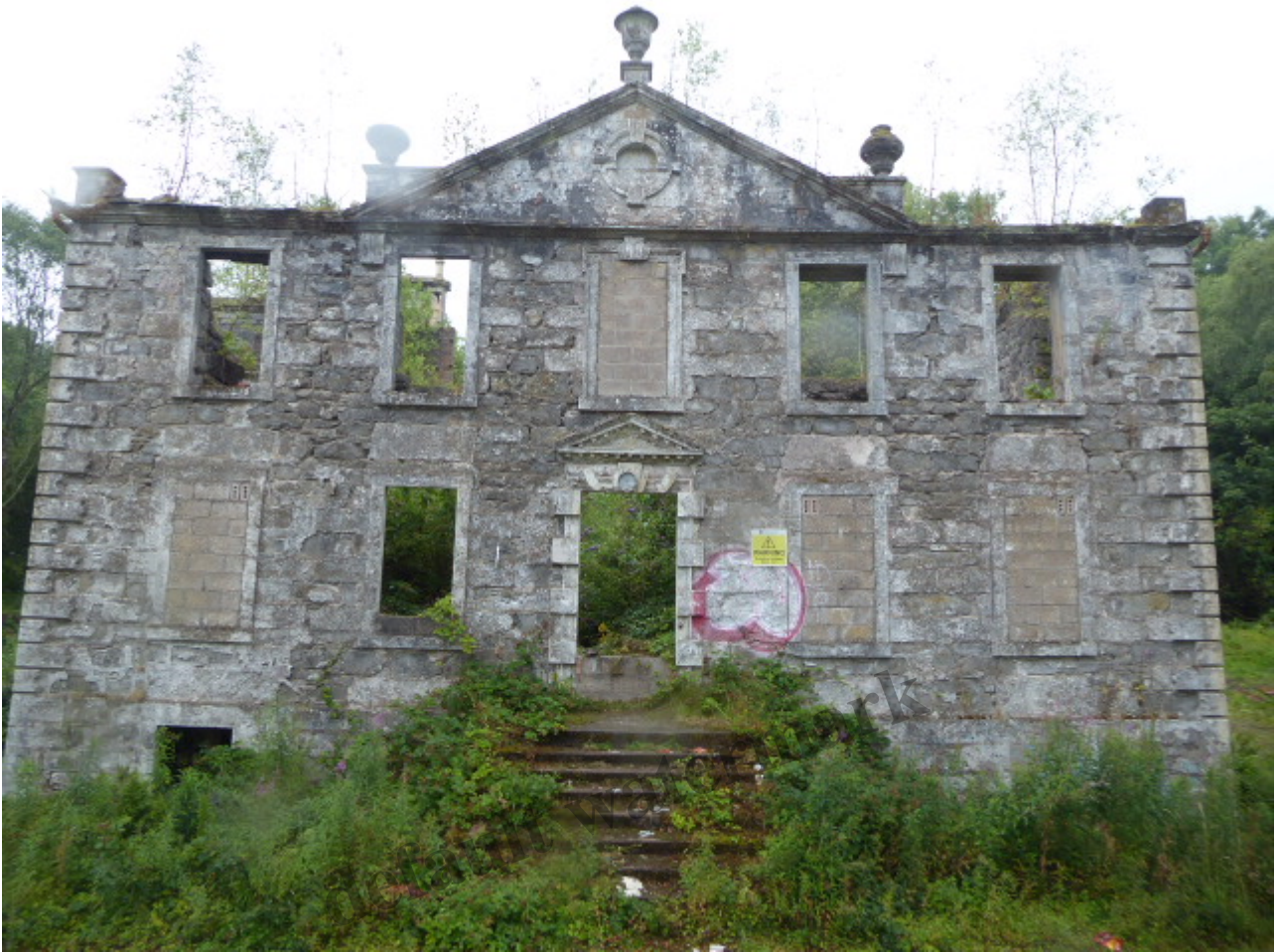
Only the outer walls of the listed Woodbank House remain
