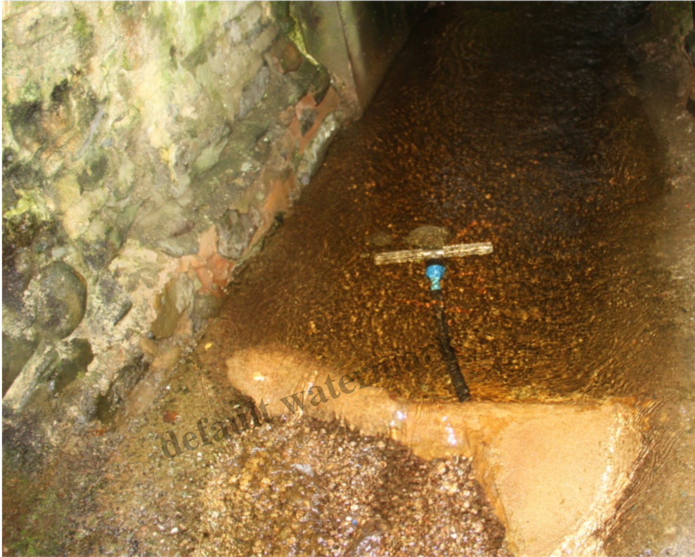
The upgraded water intake under the road bridge – photo credit Ross MacBeath
