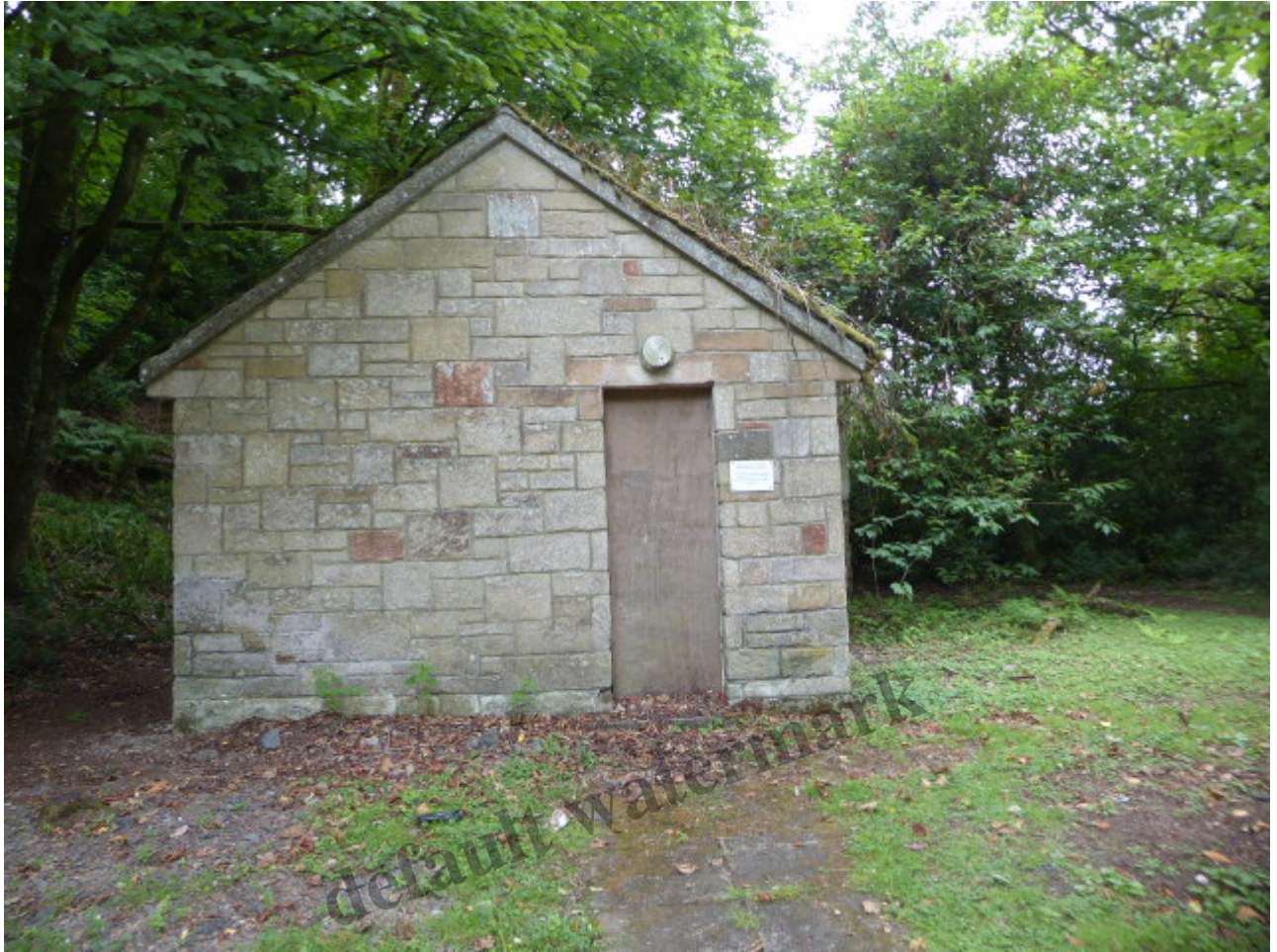
The former public toilets at Duck Bay at the south end of the car park
