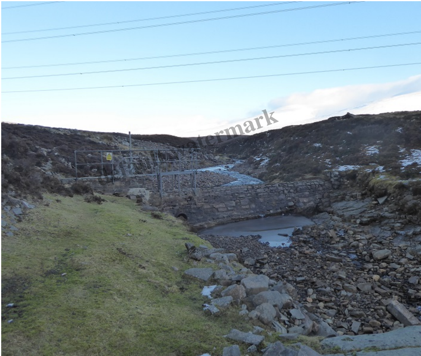
Damming of small burn under Beaully Denny powerline opposite Dalwhinnie
