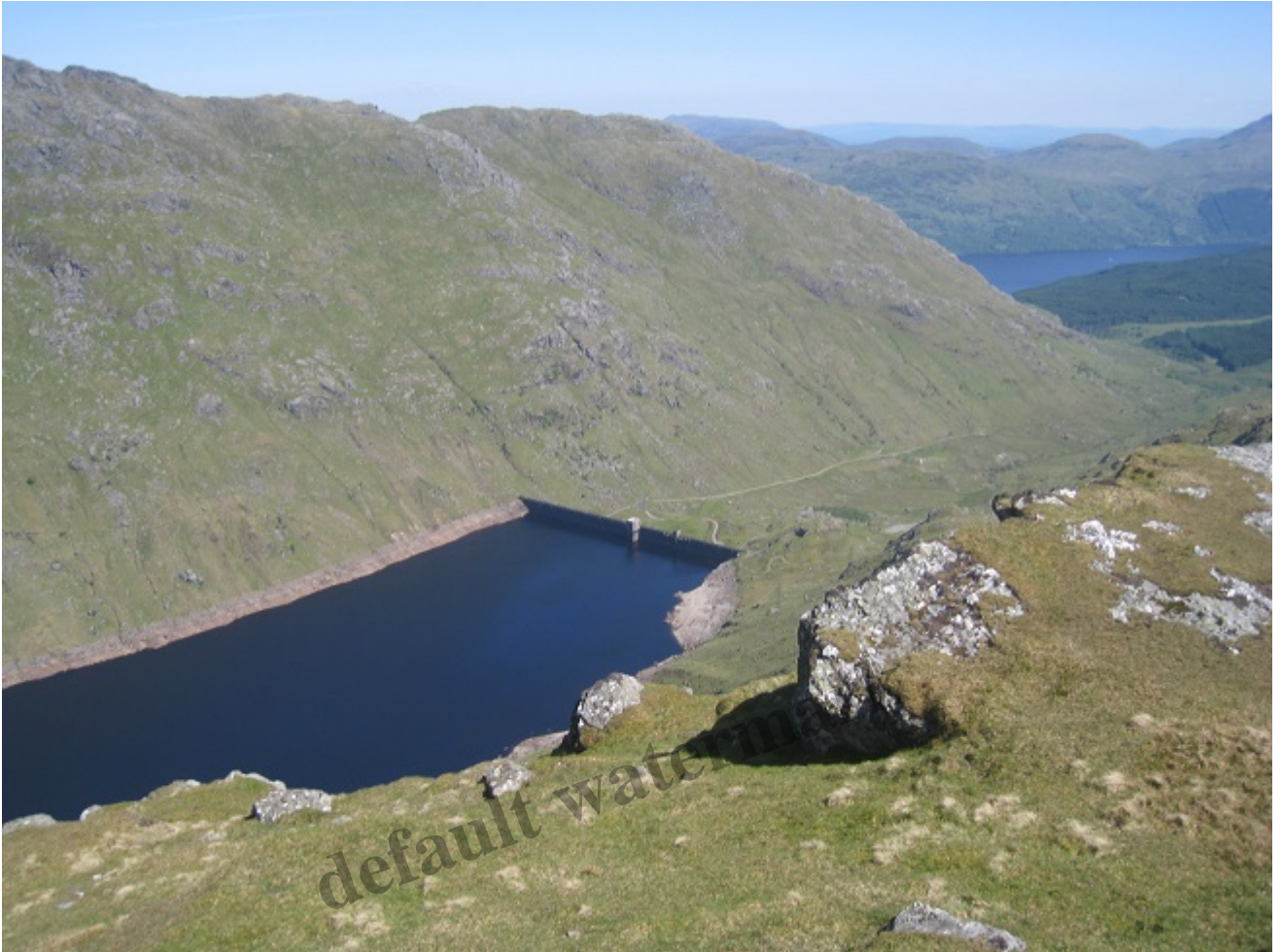
Loch Sloy from north ridge of Ben Vane in the Loch Lomond and Trossachs National Park with marked bare draw down zone characteristic of hydro lochs
