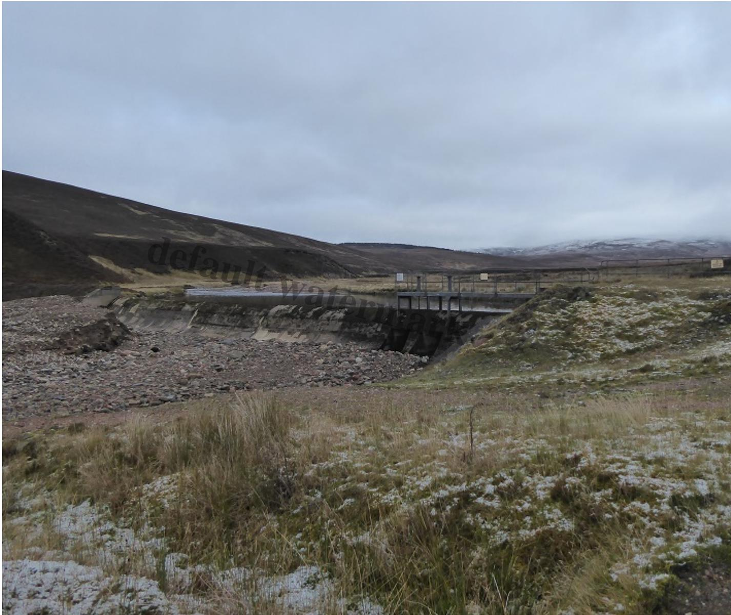
The waters from the Allt Bhran are diverted into the Tummel Hydro scheme with no water flowing from the River Tromie for much of the year
