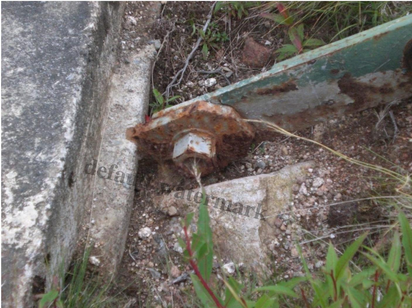
• Buried mild steel parts should be exposed and protected • photo credit Alan Bratney
