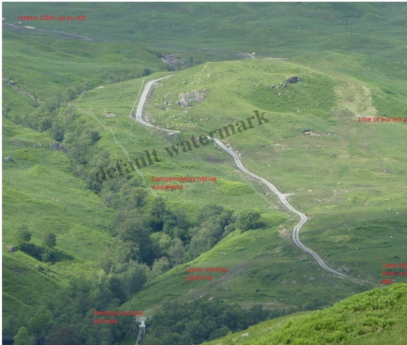
Birds eye view of central section of Eas Eonan scheme June 2018 showing the landscape impact of The line of the buried pipe has been accentuated by the dry weather.
