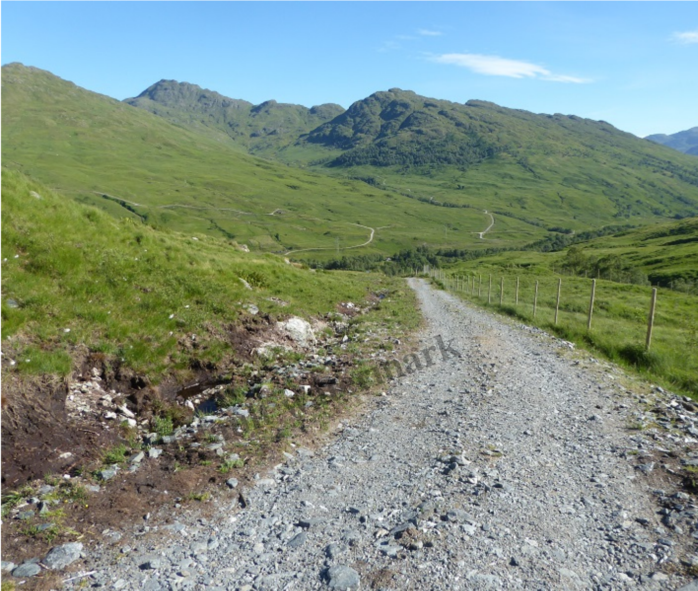
View of Derrydarroch access tracks, Allt Andoran on left, Allt a Chuillin on right, with lower section of track left middle ground. Photo taken from just above steepest section of track from one of many unmarked sections of ground now used for “estate management” purposes.
