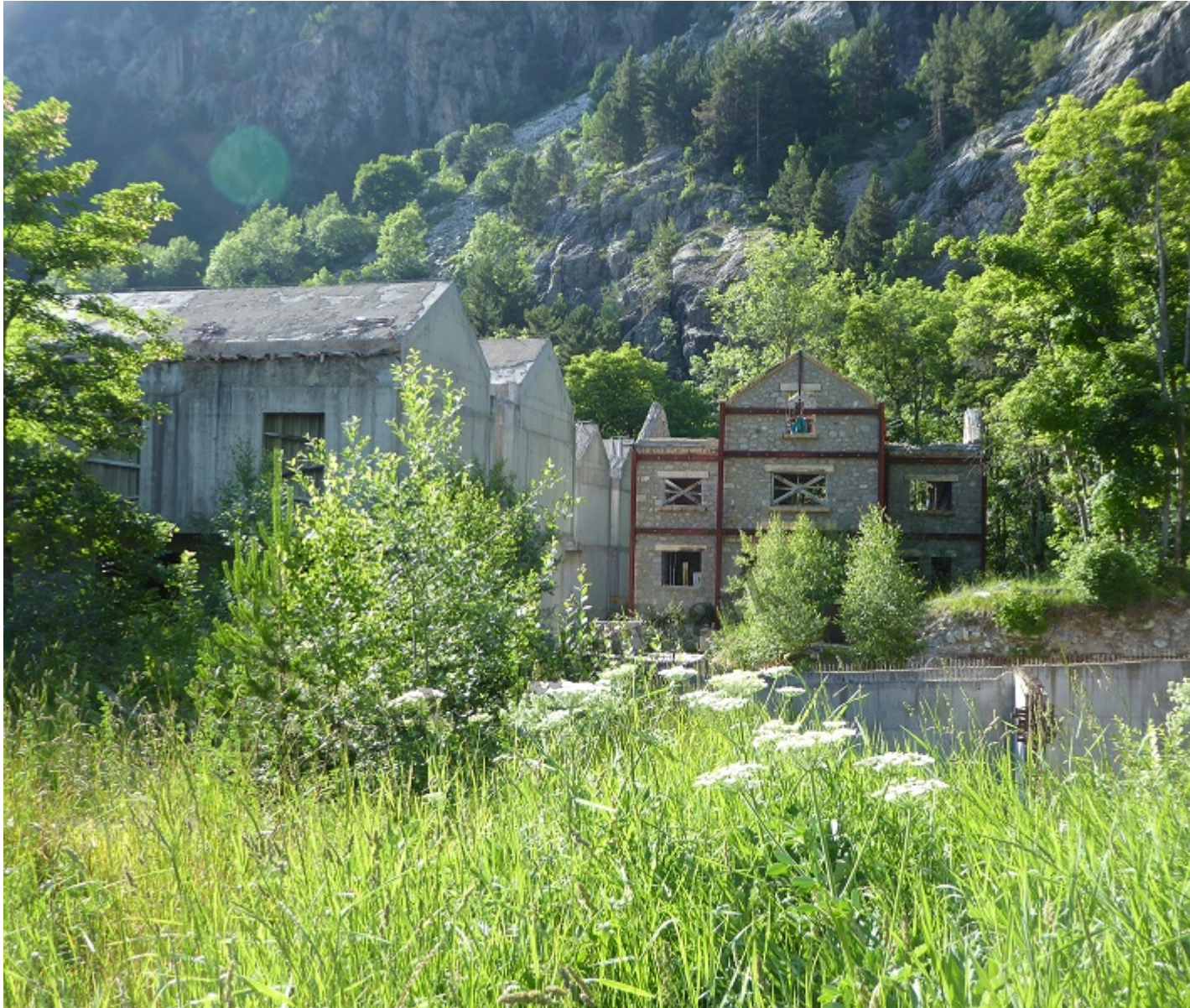
More wreckage and incompleted foundations for new buildings in foreground adjacent to the Refuge
