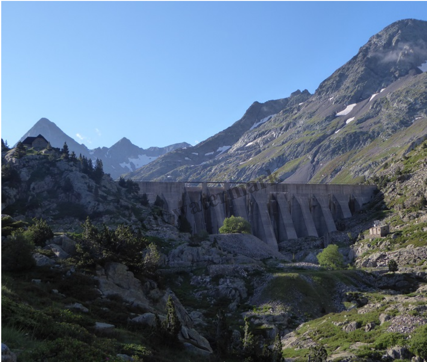
The Respomuso dam, a Spanish equivalent of Loch Sloy, but 2.5 hours from a vehicle track. Note the construction spoil below the dam.
