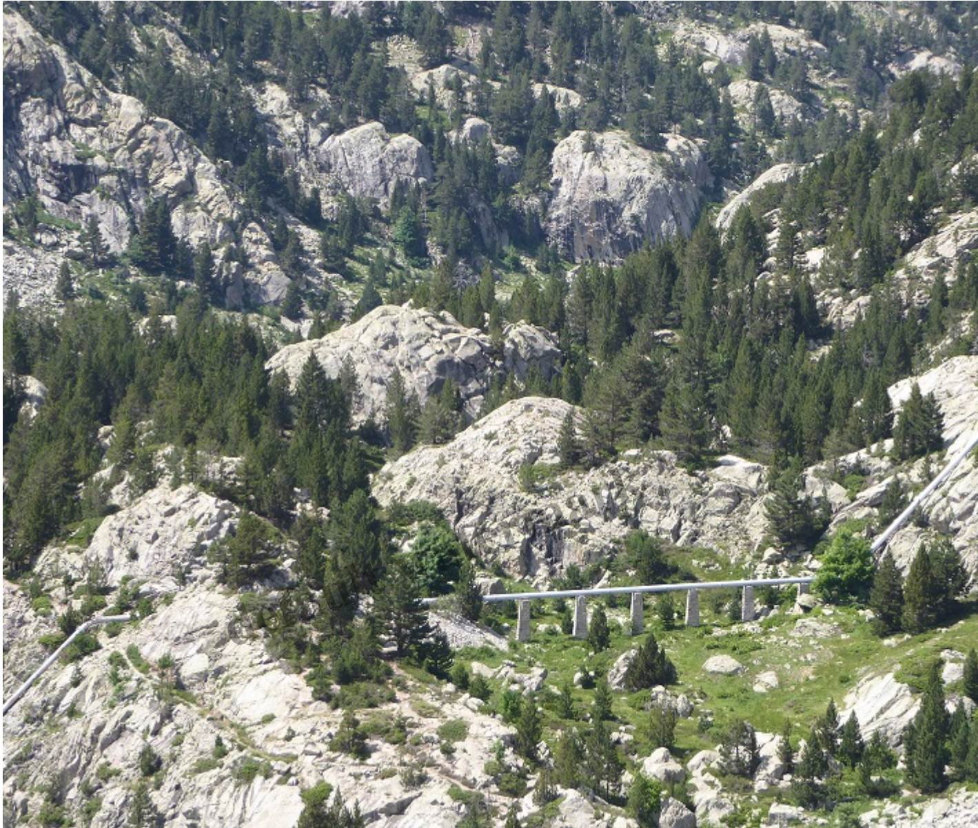
Another hydro scheme pipeline leading down to Banos de Panticosa
