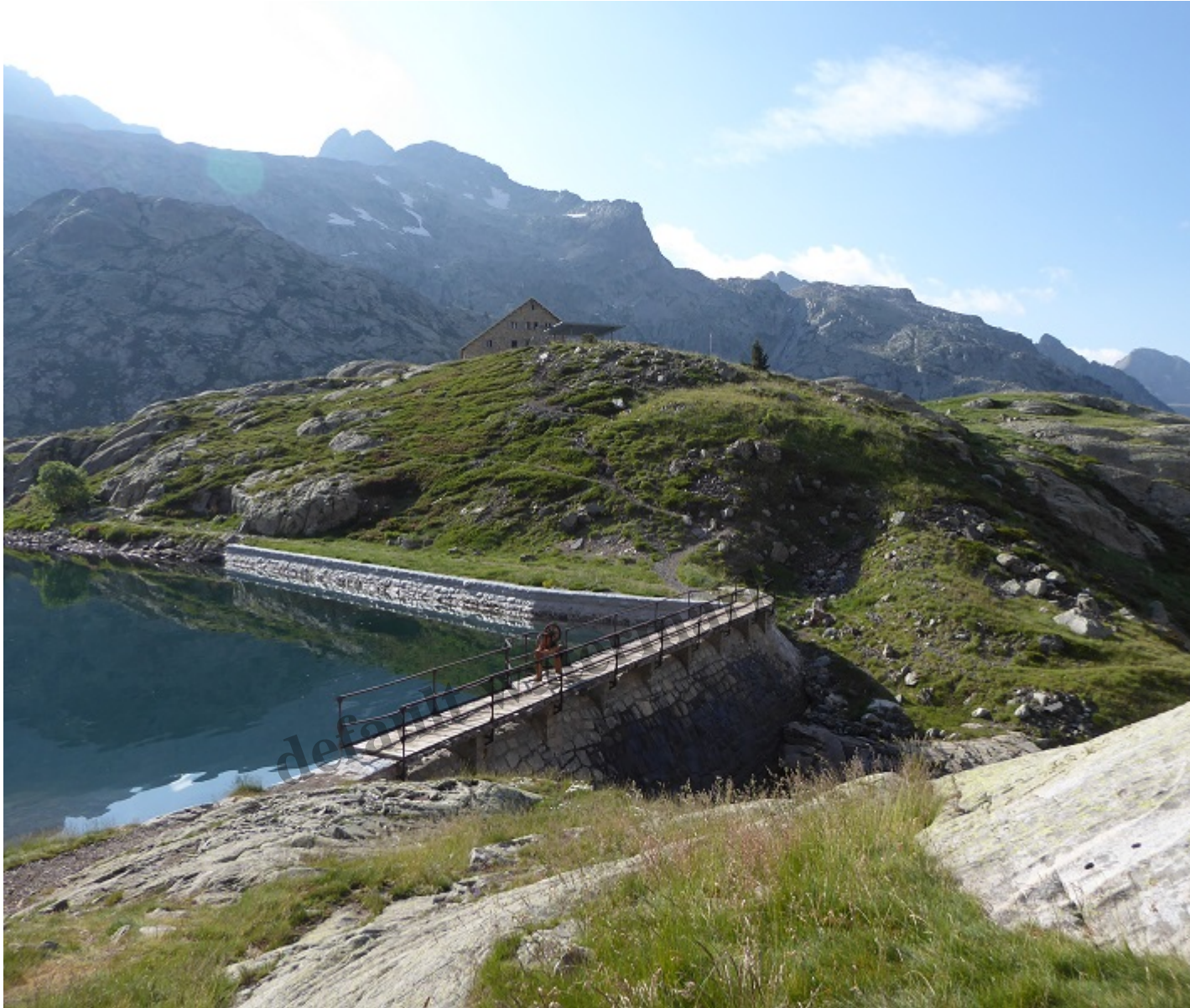
Note how both sides of the (newly extended) dam walls at the Embalse de Bachima Alto, by the new Hut on the GR11, have been faced with stone
