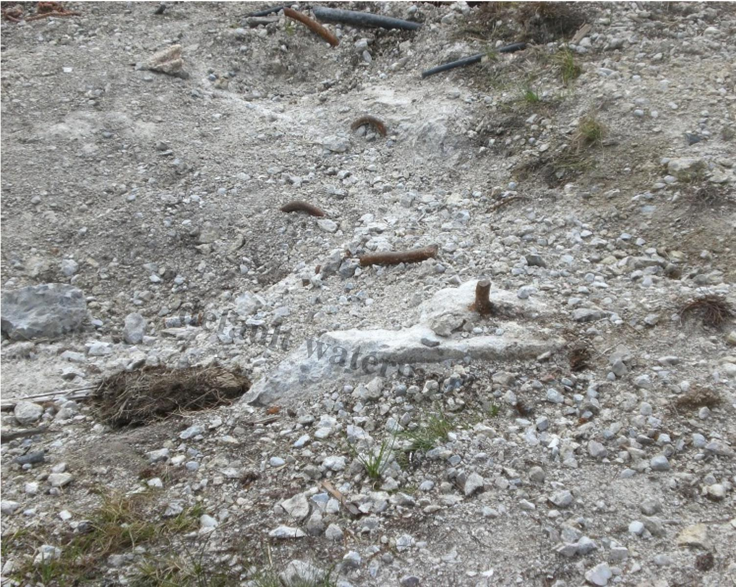
Very dangerous reinforcing metal rods that have been left protruding from the concrete.
