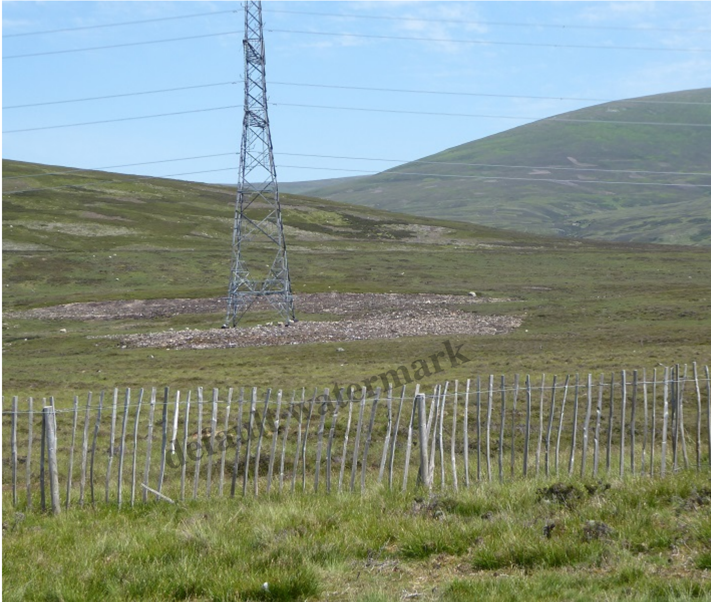
Pylon across A9 from Dalwhinnie
