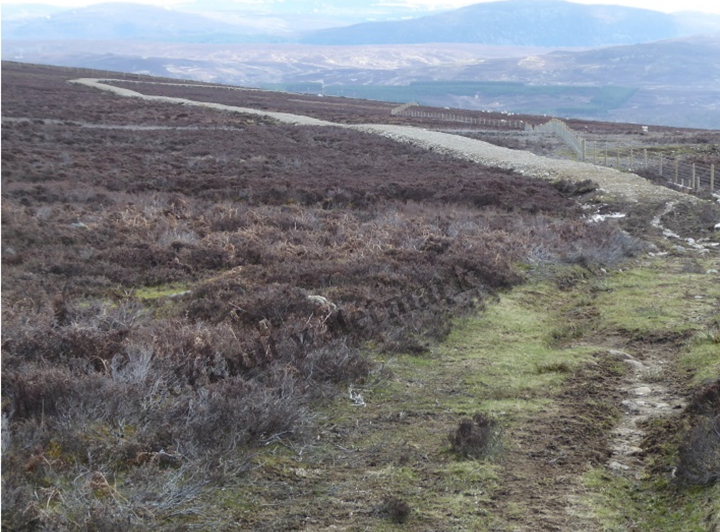
The top section of the new track along the Allt Mhor
