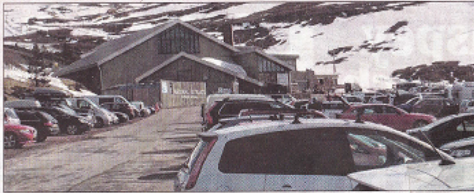
CHARGING DRIVE: Coire Cas car park towards the end of last winter with the Base Station and the Day Lodge in the background.
