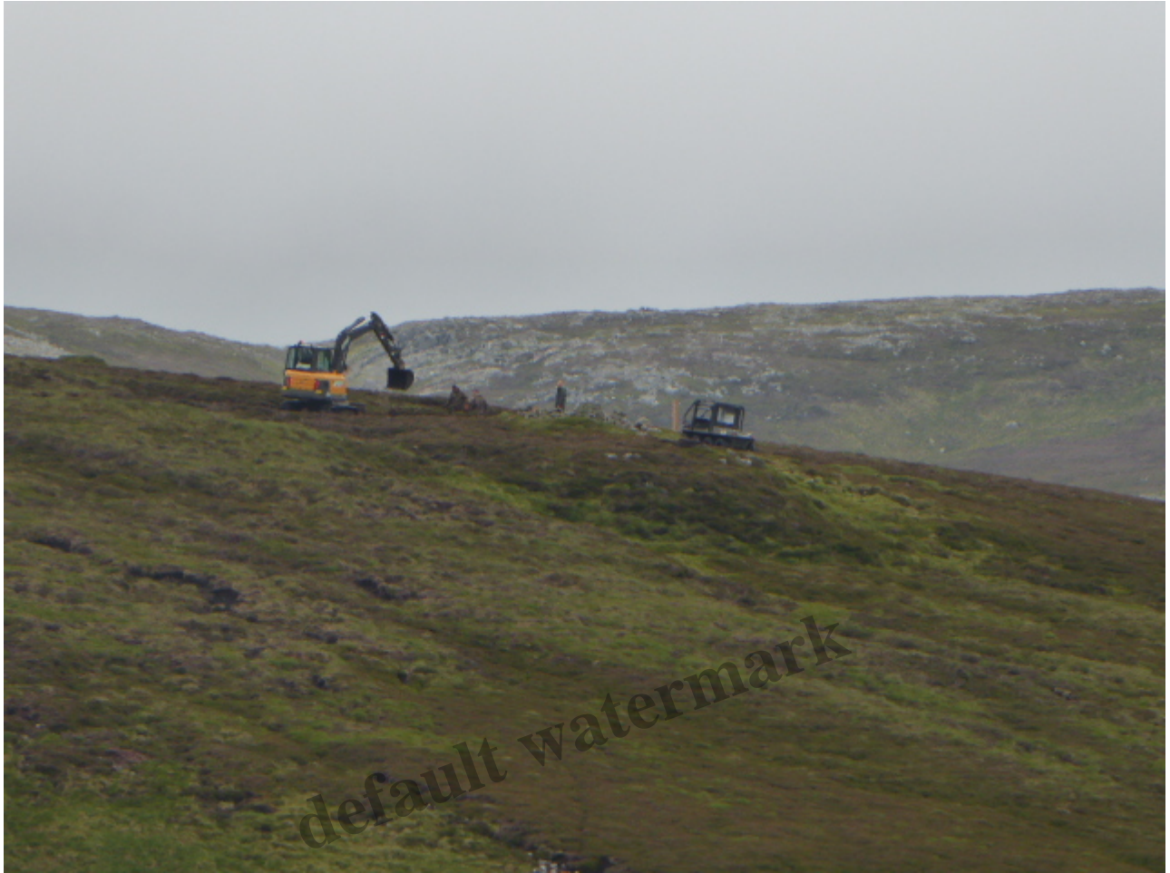
Telephoto shot of digger working
