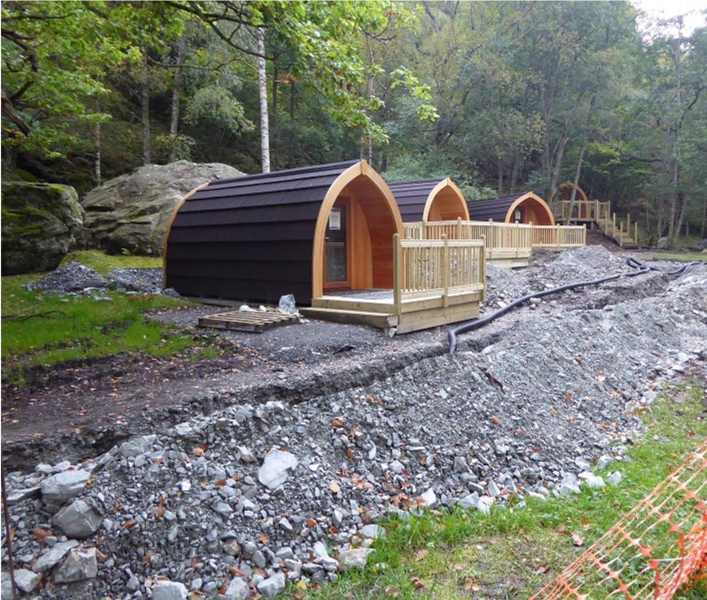
The Eco Camp under construction last year
