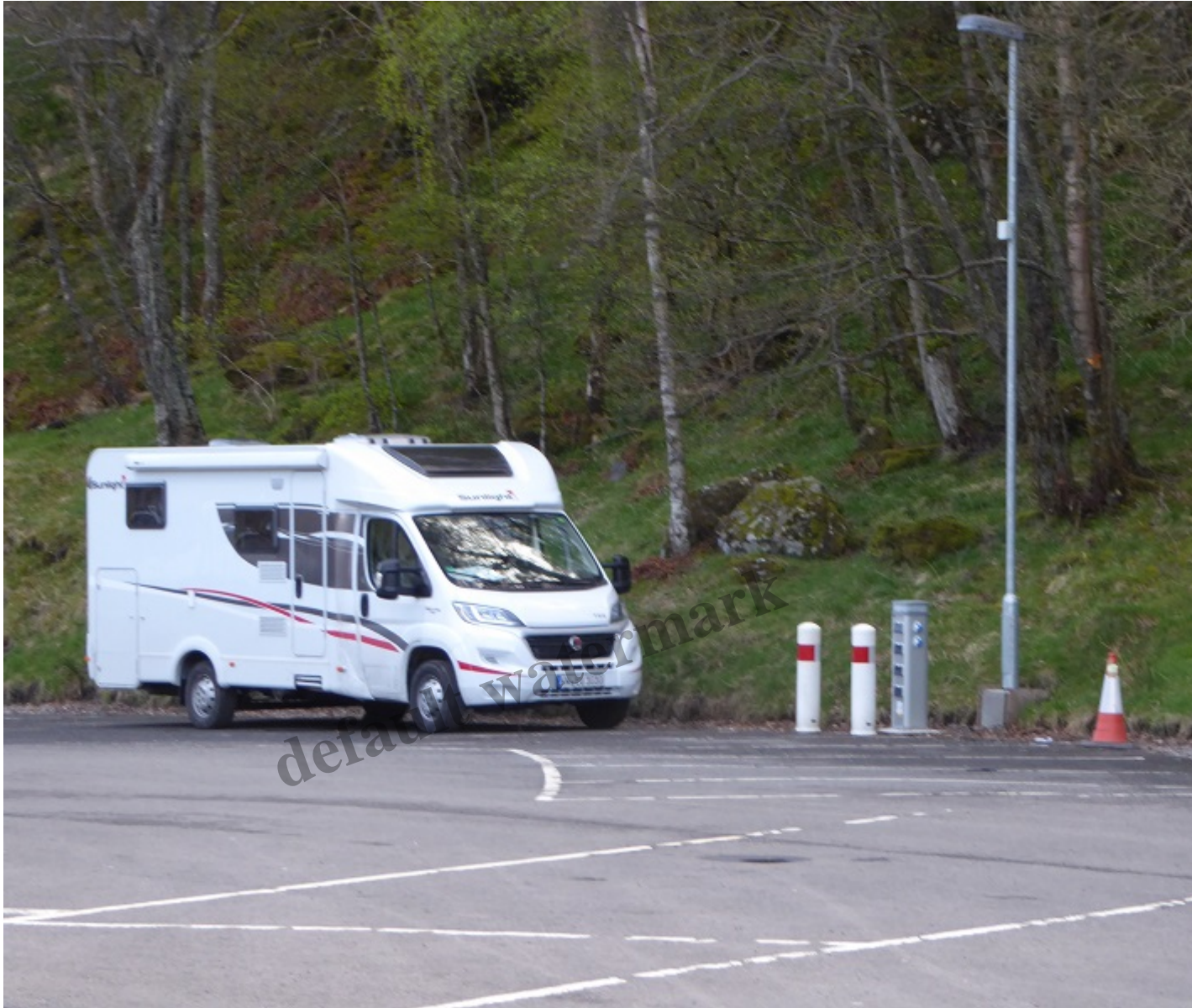
Powerpoints for campervans in the main car park
