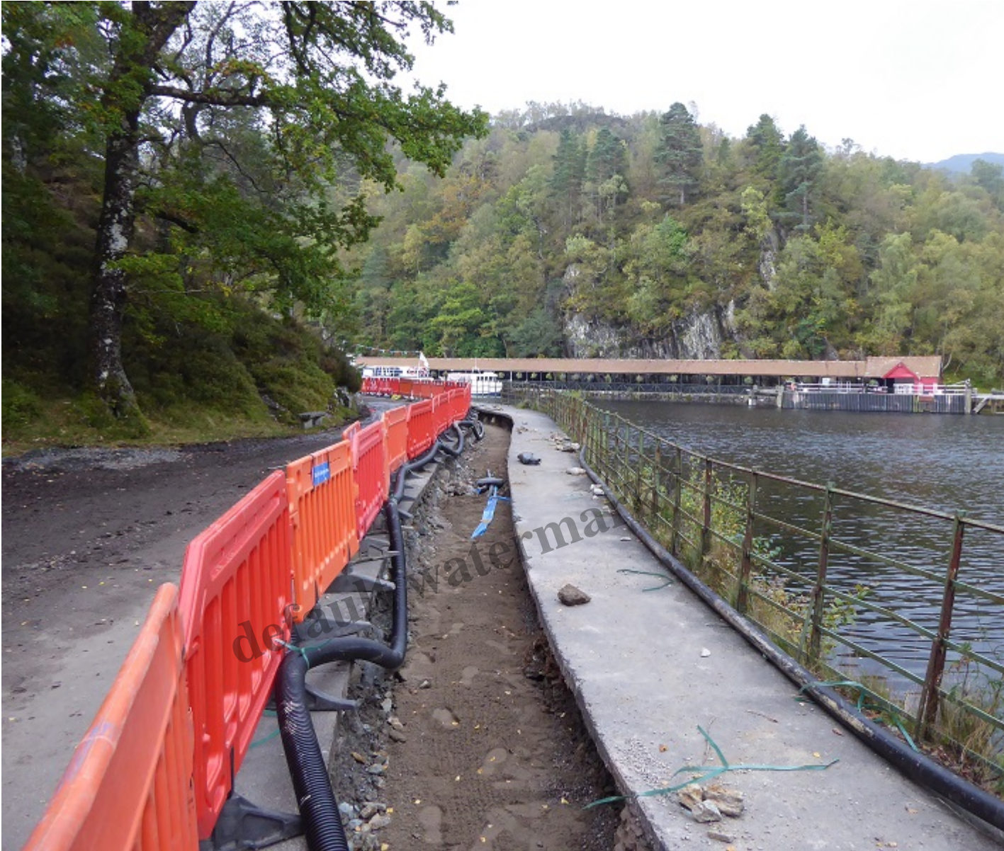
Water supply and utilities connection under construction last year
