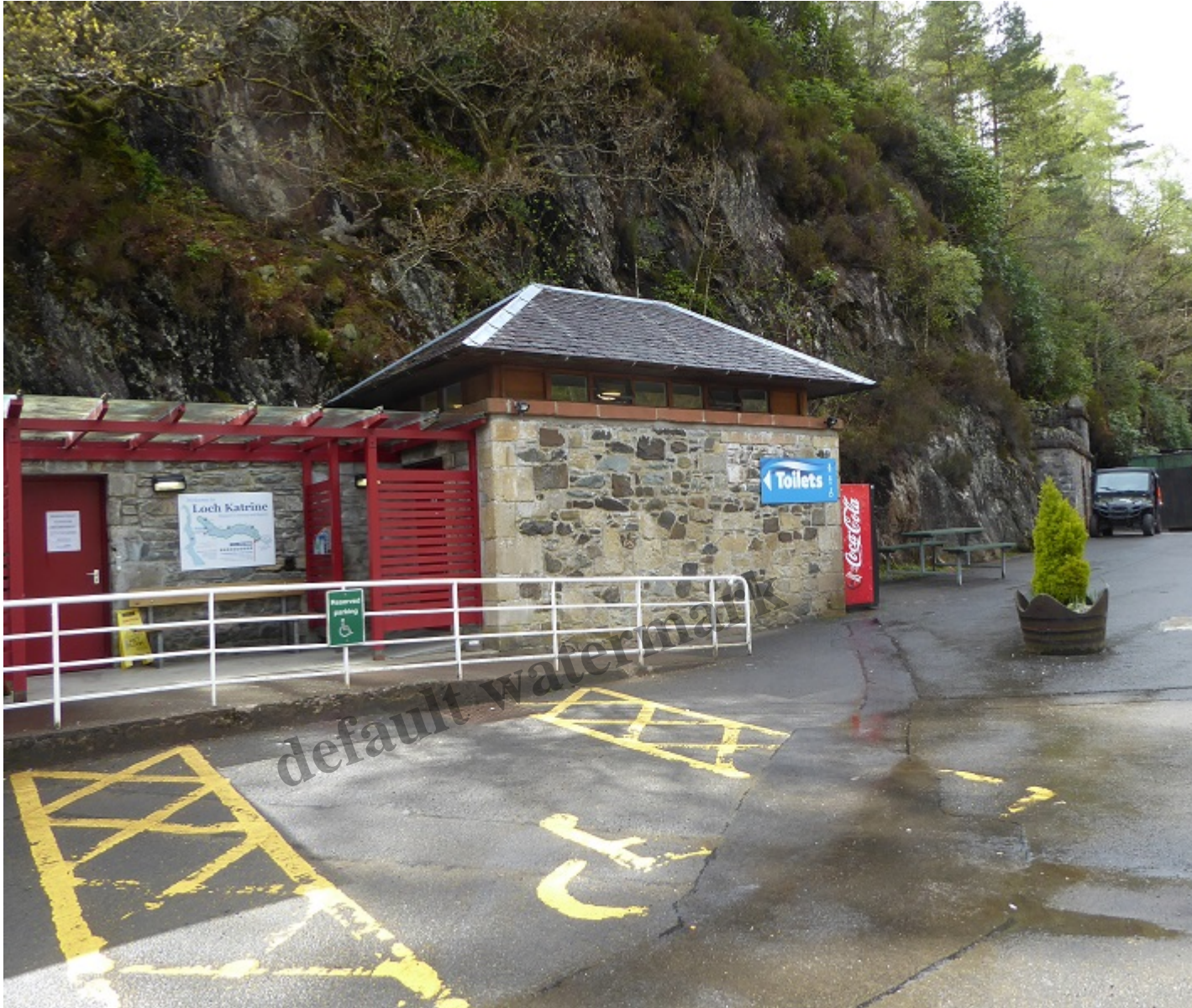
The car park toilet block now includes a shower
