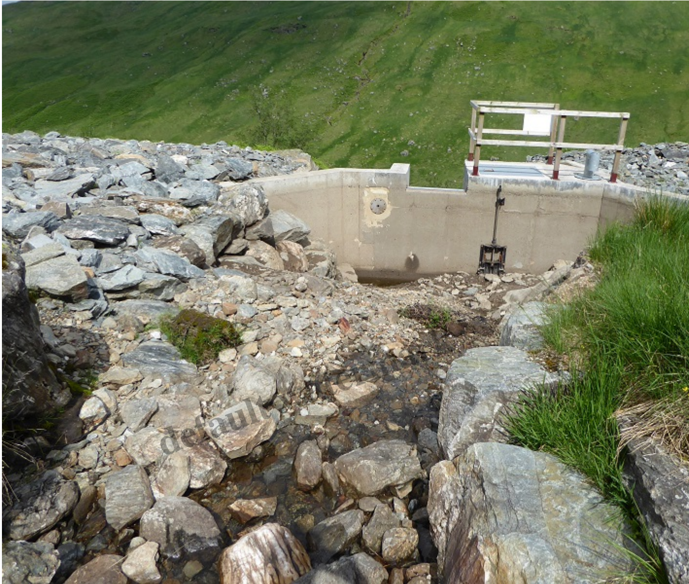
The third intake from above with flowing water visible in the foreground
