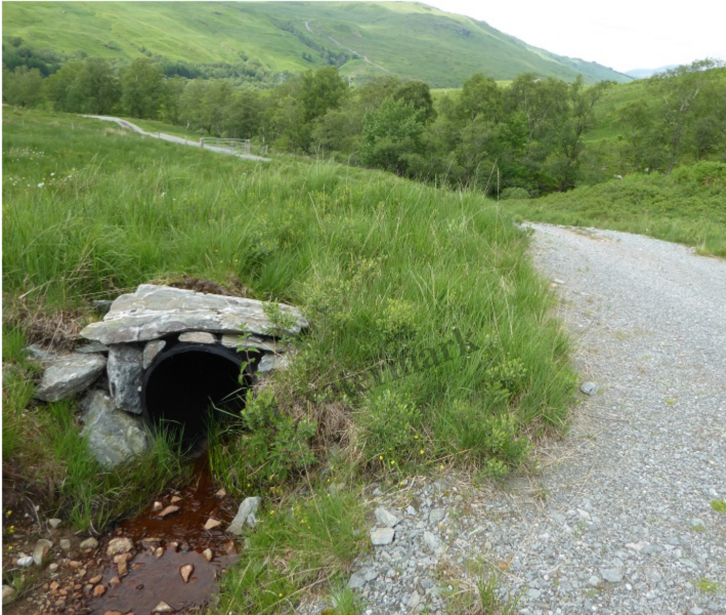
The lower section of the track along the Allt a'Chuillinn
