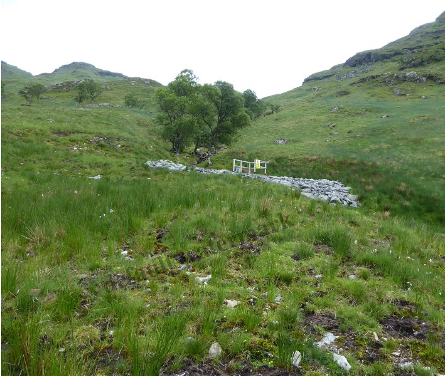
View along the pipe which leads down from the second intake
