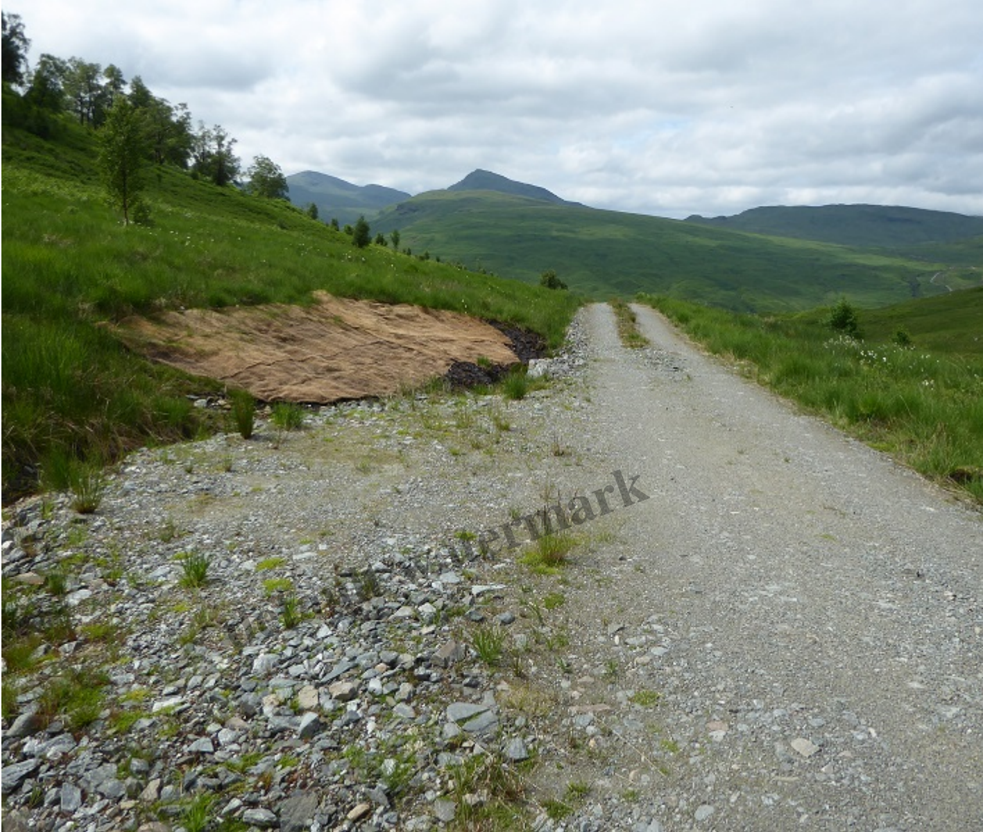
Matting being used to try and restore areas of bare peat
