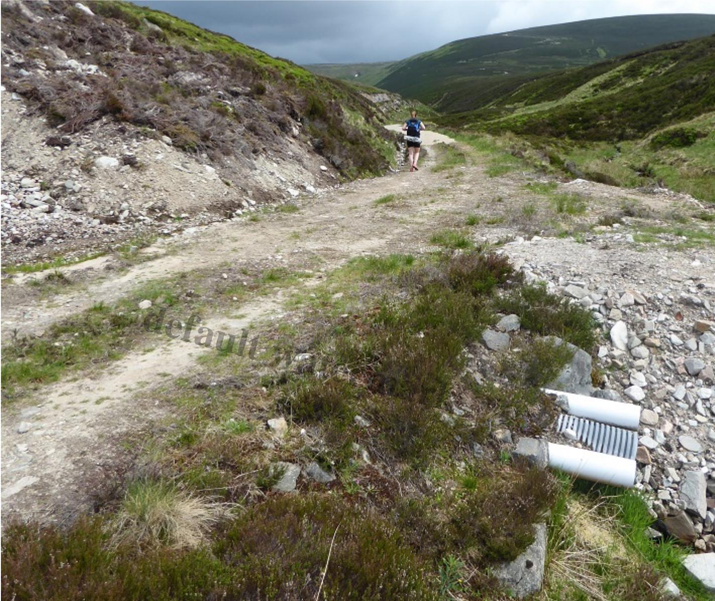
Note the attempted and partial restoration of the slope (top left) marked by the dead heather and how the path on the right is likely to erode straight into the burn
