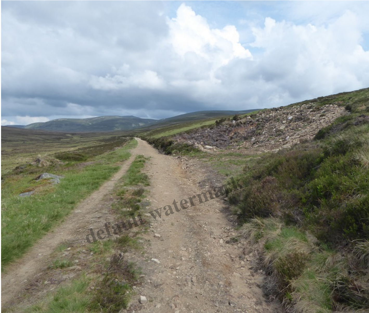
The start of the first section of upgraded track, with newly worked borrow pit on right
