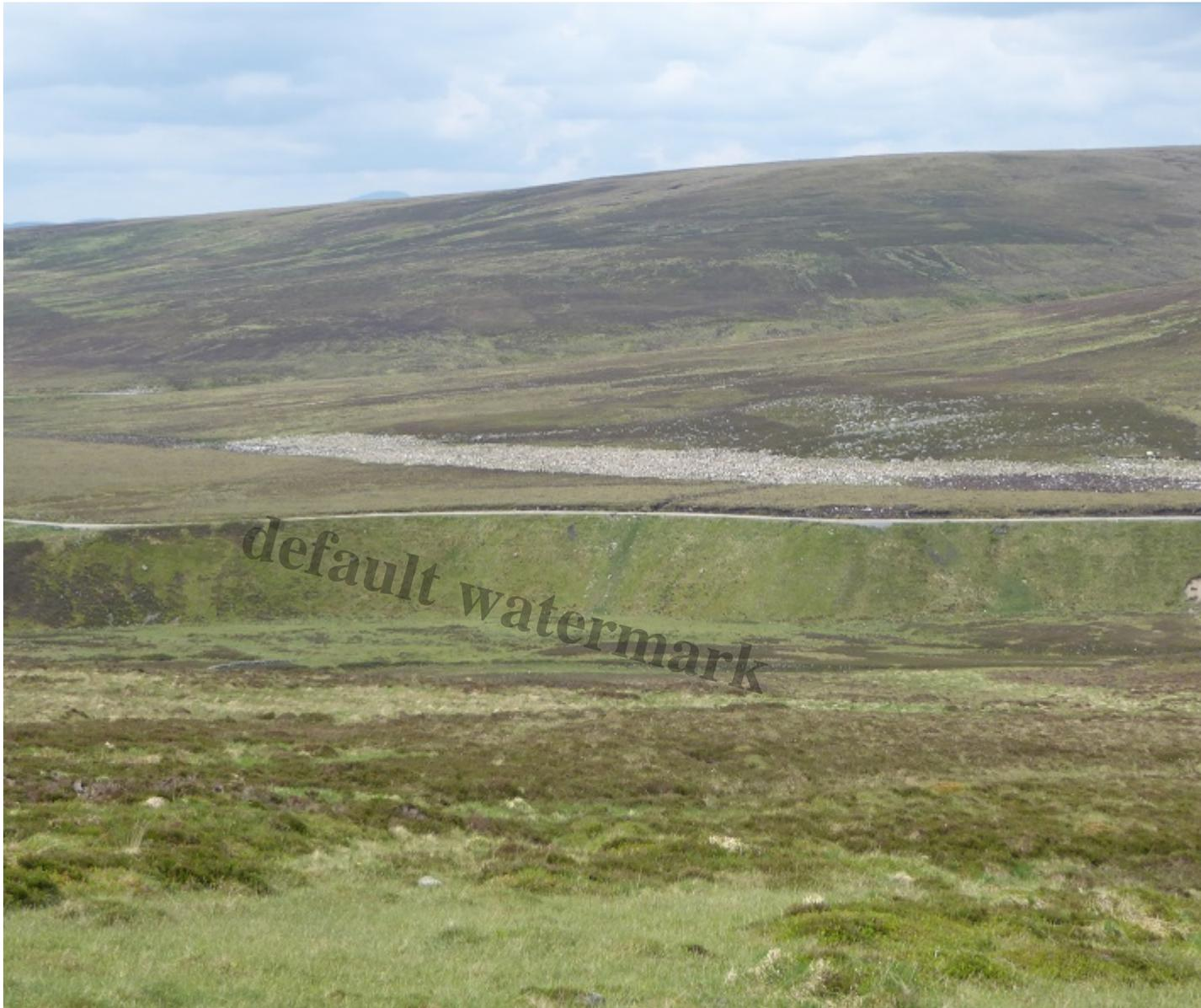
The worst section of the Bruar pipeline restoration where boulders, which were previously covered by heather, have been left on the surface forming a great landscape scar. At the far left end of the scar you can see how the restoration should have looked and on the middle right you can see where peat (the dark line) has been stored for restoration purposes has been used to cover some of the scar.
