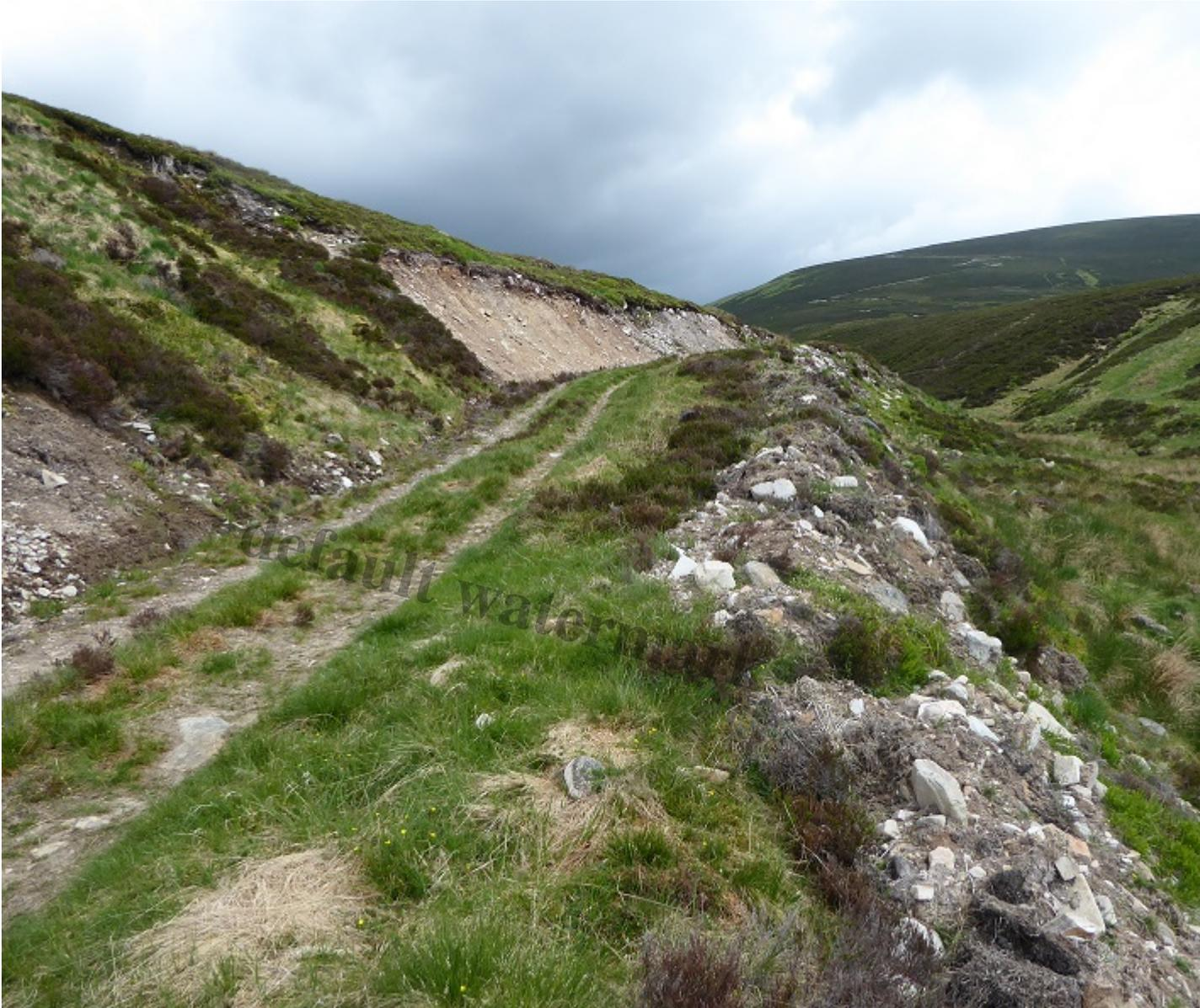
It is not clear why soil and vegetation has been dumped alongside the right of the track here when it has been used to restore some of the bare banks
