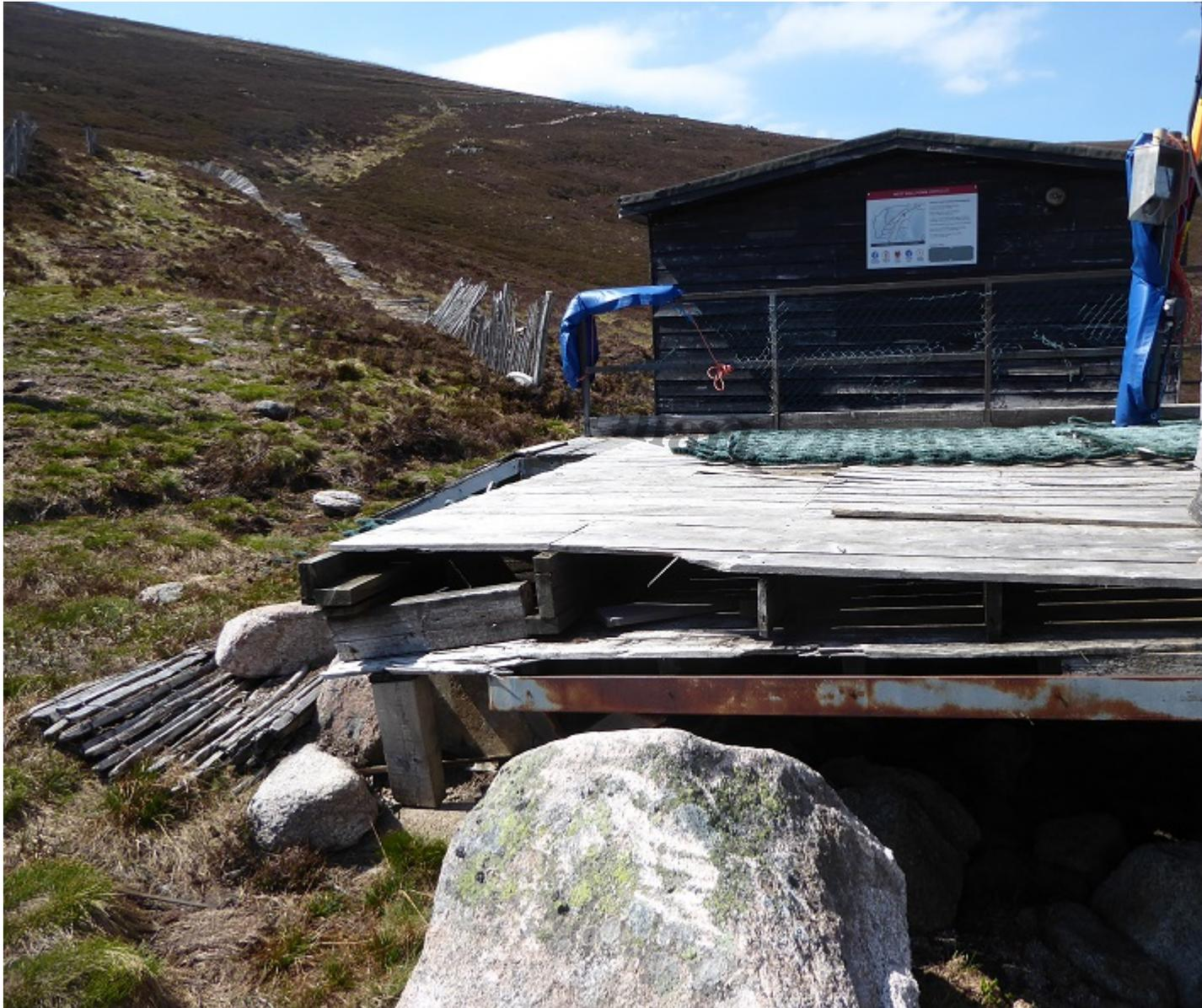
The West Wall poma base, in urgent need of repair, with electricity sub-station and collapsed snow fence behind on 26th May 2018
