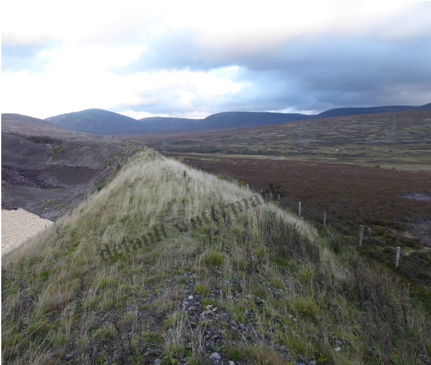
View east along the southern bund which screens the quarry from Dalwhinnie. A9 and Meall Cuaich
